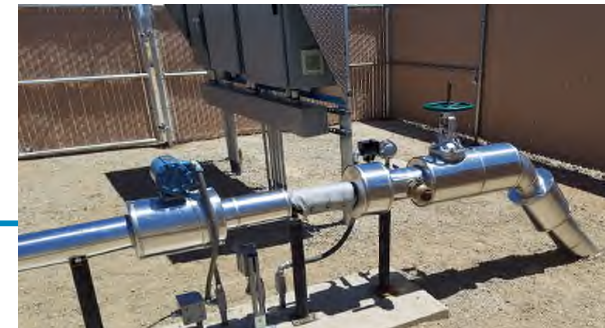
New extraction wells for plume containment and contraction
