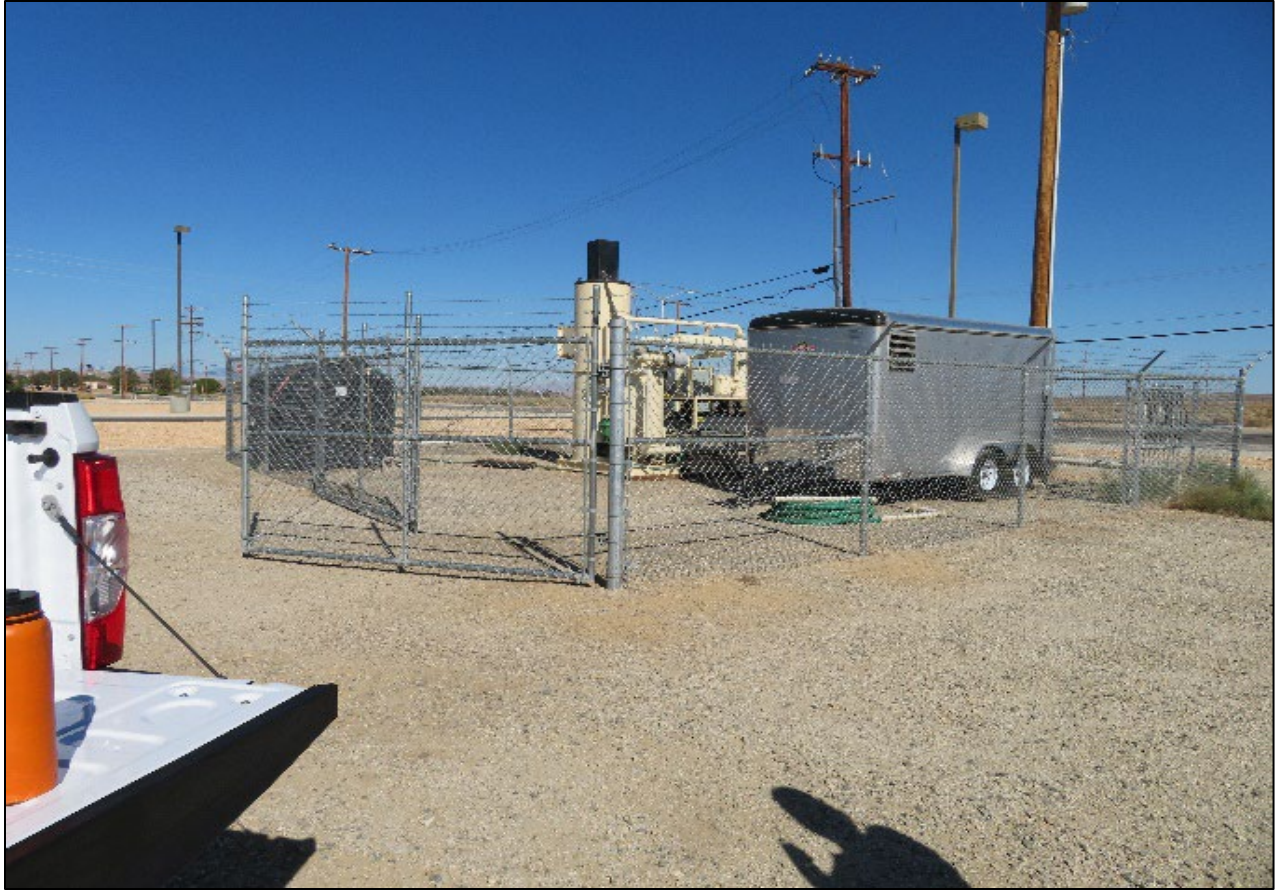
Photo 3.1: View of the air sparge (AS)/soil vapor extraction (SVE) system at Site 297. The SVE system (beige system in background) was upgraded with a new Mako Industries Inc. (Mako) thermal/catalytic oxidizer SVE system in June 2021. This replaced the repurposed Baker Furnace SVE system that was installed onsite in 2019.
