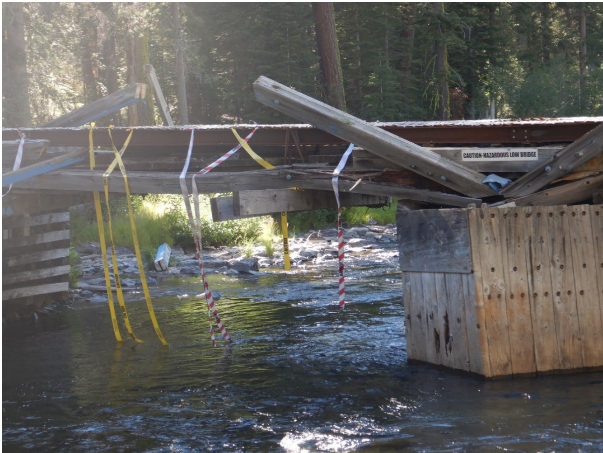
Figure 2.1—Photo of the collapsing bridge span with caution tape used to warn Truckee River recreators
