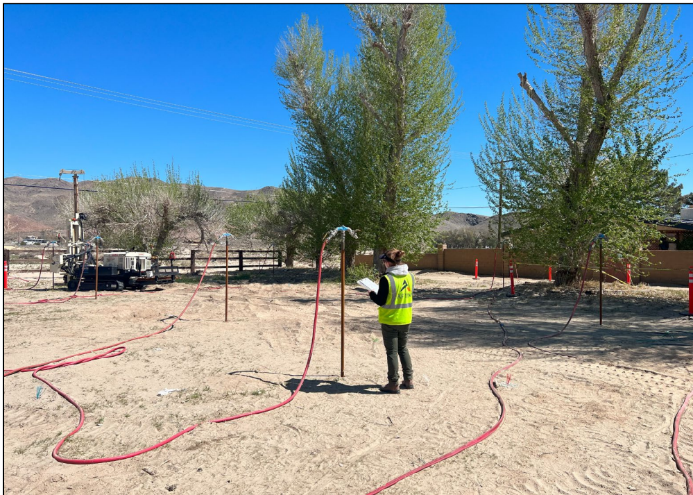
Photo 5.7: Field technician checking connections and making note of injection operations in the “garden area.” Photo facing northeast.
