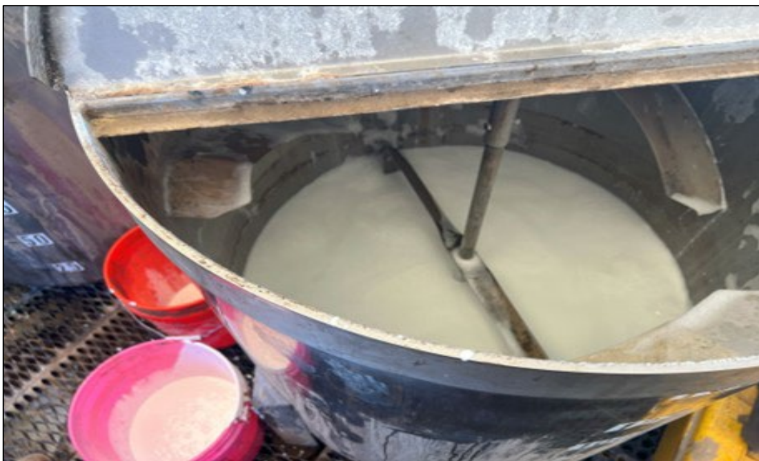
Photo 5.2: The EVO mixing in a 55-gallon steel drum prior to injection
