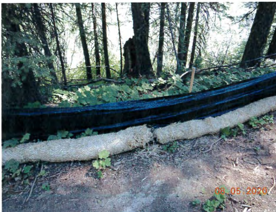
Photo 11. Downslope perimeter sediment control BMPs.
