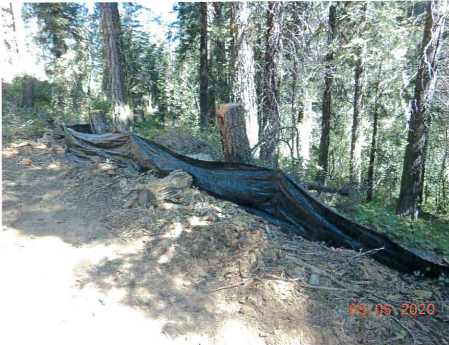
Photo 10. Downslope perimeter sediment control BMP.
