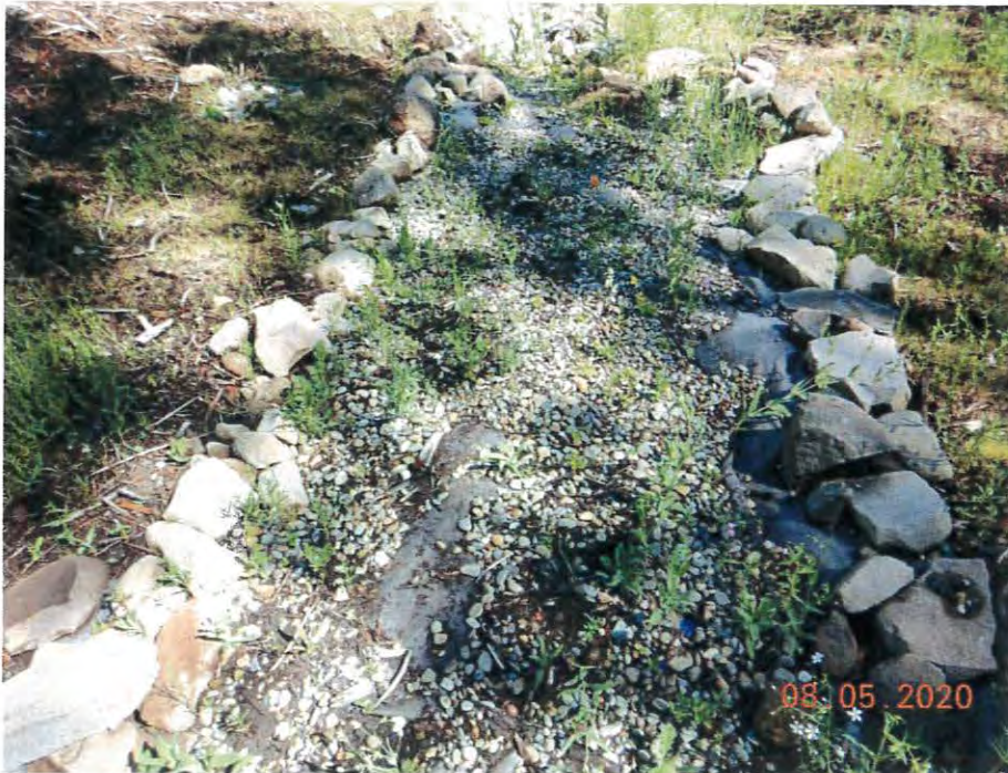
Photo 16. Modified watercourse: straightened, lined with geotextile, covered with gravel, bordered with cobbles.
