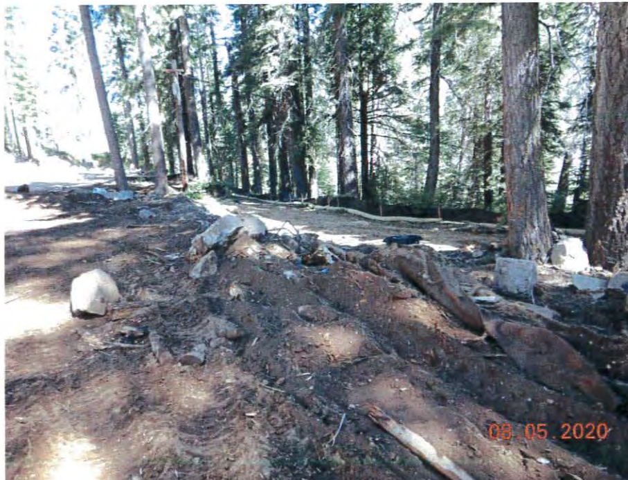
Photo 7. Windrowed soil and rock, downslope perimeter BMPs
