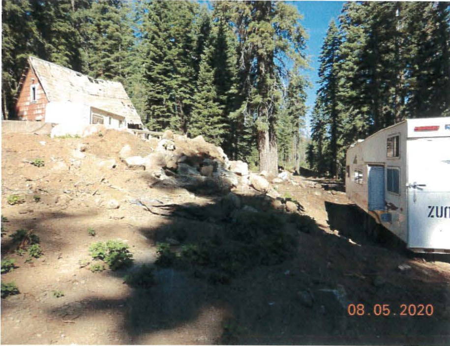
Photo 4. Stockpiled soil and rock.
