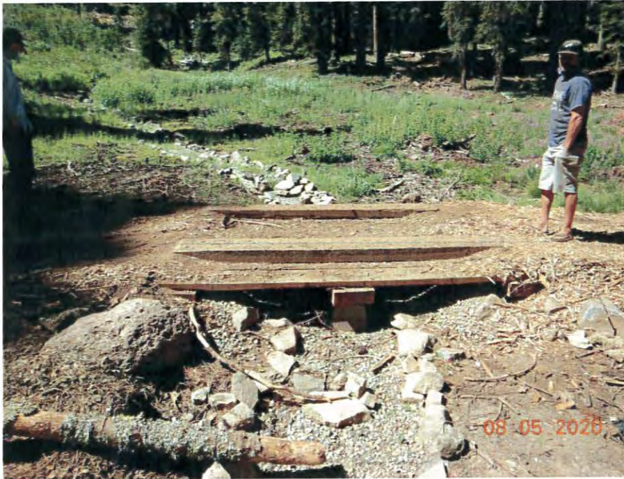
Photo 14: Permanent watercourse crossing.
