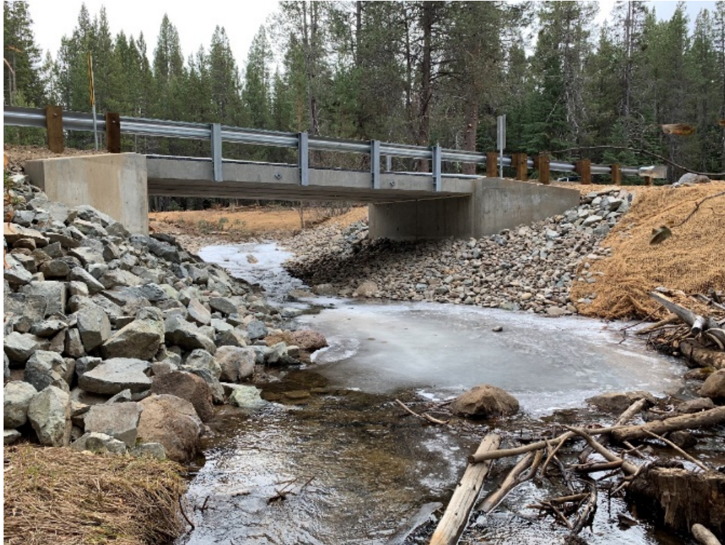
Photo 1: Completed Saxon Creek Bridge
