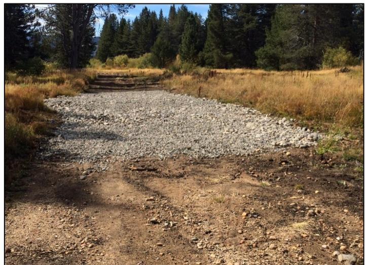
Photo 4 – Rock cobble rolling berm constructed along a Project access road in October 2018, as part of the 2018 Implementation and Monitoring Plan.
