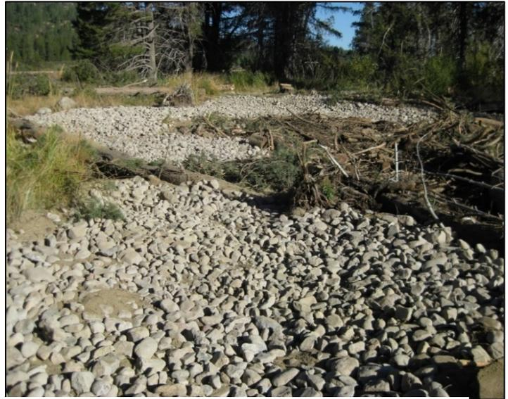
Photo 2 – Sand bag berm removal and content stabilization conducted in September 2018, as part of the 2018 implementation and Monitoring Plan.
