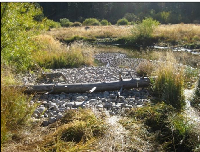
Photo 3 – Upper Truckee River bank stabilization materials placed in September 2018, as part of the 2018 Implementation and Monitoring Plan.
