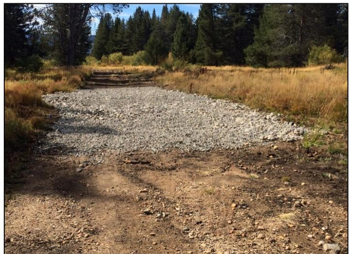
Photo 4 – Rock cobble rolling berm constructed along a Project access road in October 2018, as part of the 2018 Implementation and Monitoring Plan.
