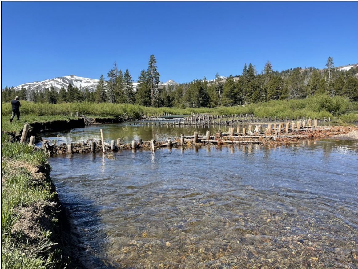
Photo 6.1: Beaver dam analogues recently installed in the river as part of the Faith Valley Meadow Restoration Project, one of the restoration projects expected to reduce nutrient and sediment inputs into the river, June 2024. The Implementation Summary Table below includes an update on restoration projects under the implementation action titled Stream Restoration on the WFCR.
