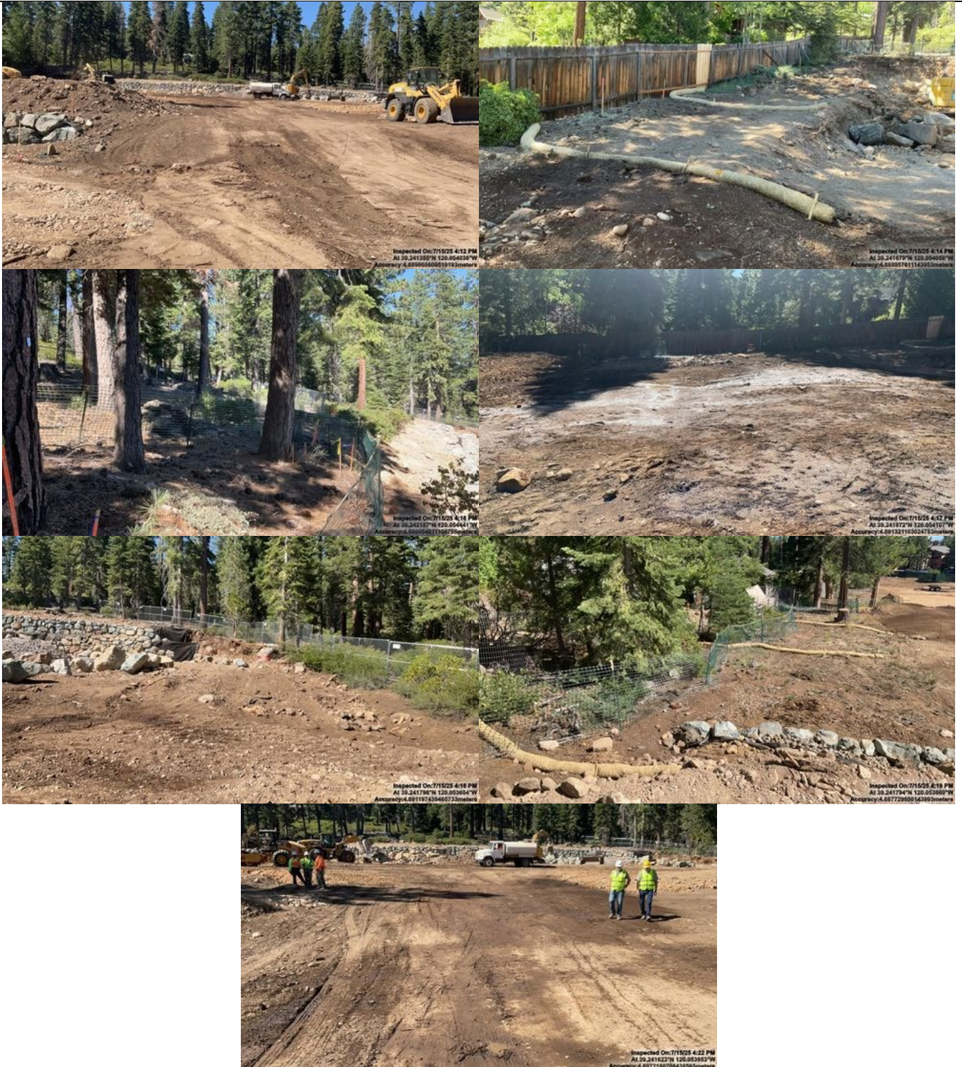
Photos 17-23: Stop 3: Check Dams and Run-on Controls, North Excavation, and Dust Suppression Water
