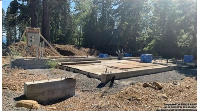
Photos 14-16: Stop 2: Mulch Stockpile and Retaining Walls
