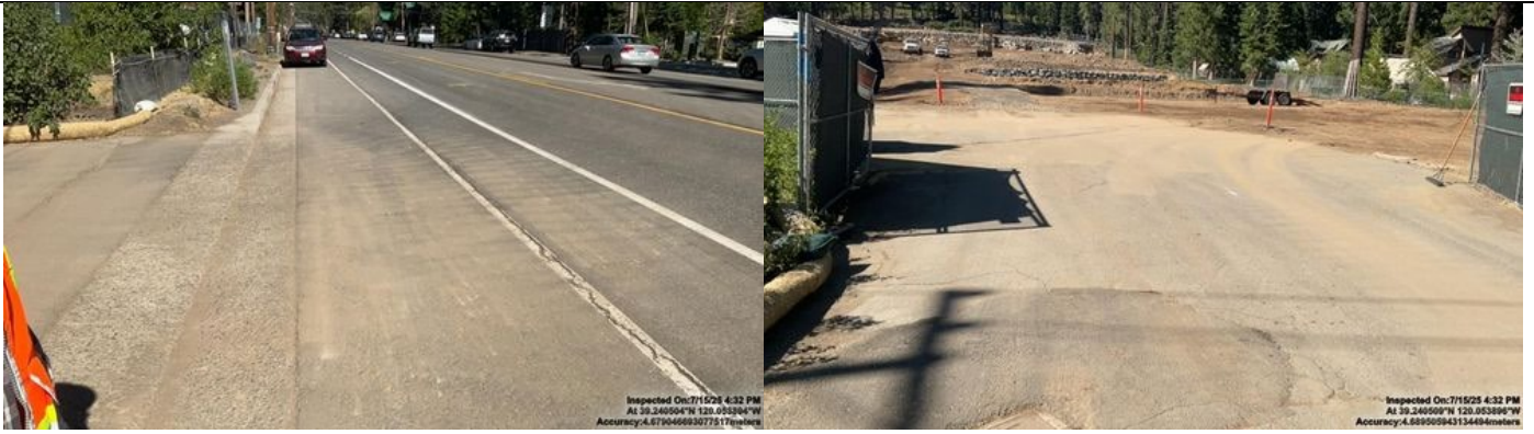
Photos 24-33: Stop 4: Equipment Storage Area, Construction Entrance, and Site Frontage along Highway 28
