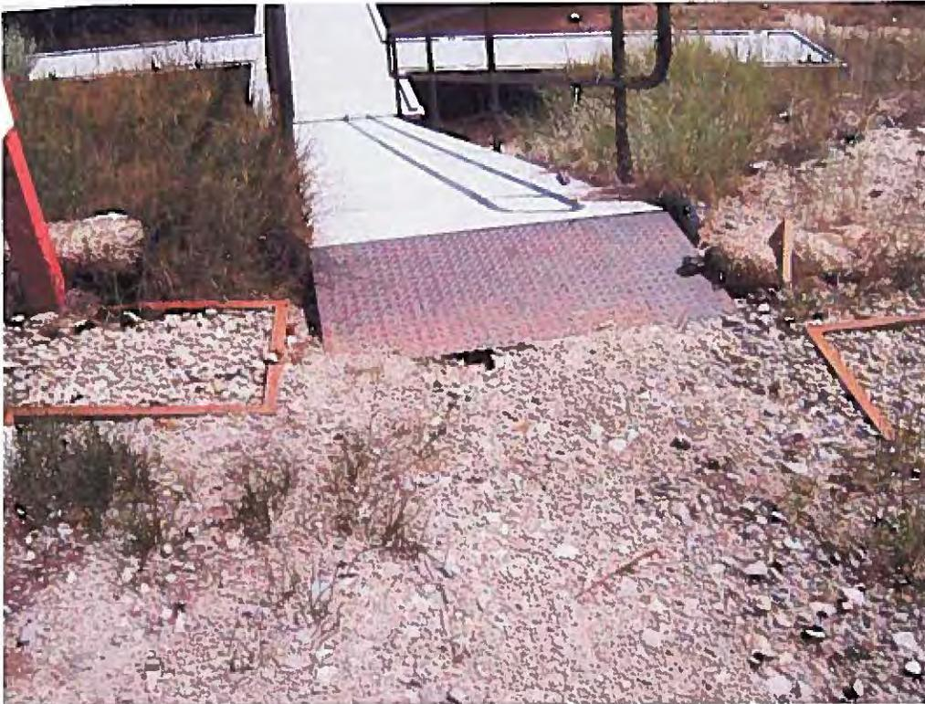
**Photograph 17 - 3rd ramp west from office, facing south. A rill has formed beneath the metal plate, creating a threatened discharge of sediments into the marina. No fiber rolls or other BMP exists to prevent runoff from flowing down this area and causing bank erosion.**
