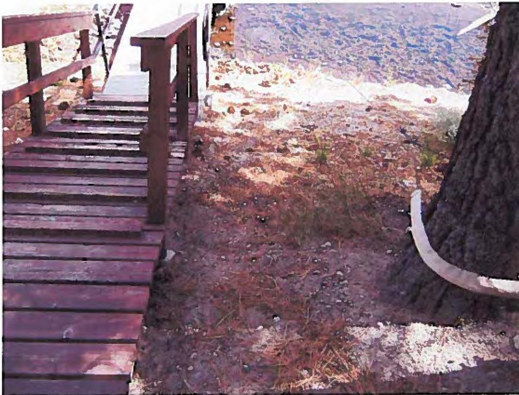
Photograph 24 - Close-up of the west side of the 4<sup>th</sup> walkway shown in Photograph No. 20. Evidence of erosion can be observed.
