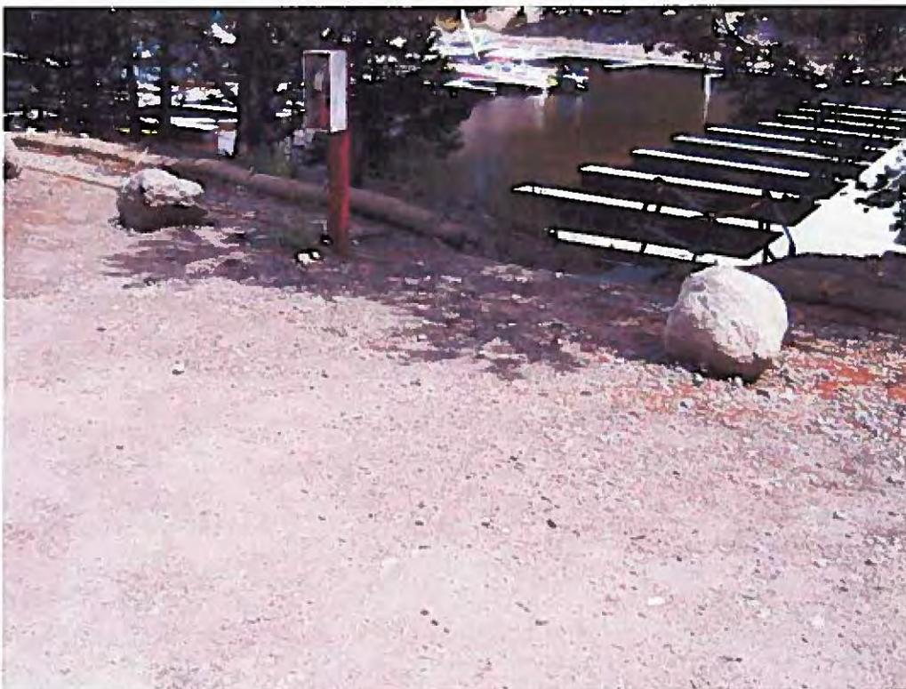
**Photograph 08 - Second ramp west of office, facing southeast. Fiber rolls do not prevent runoff from going down ramp and into marina.**
