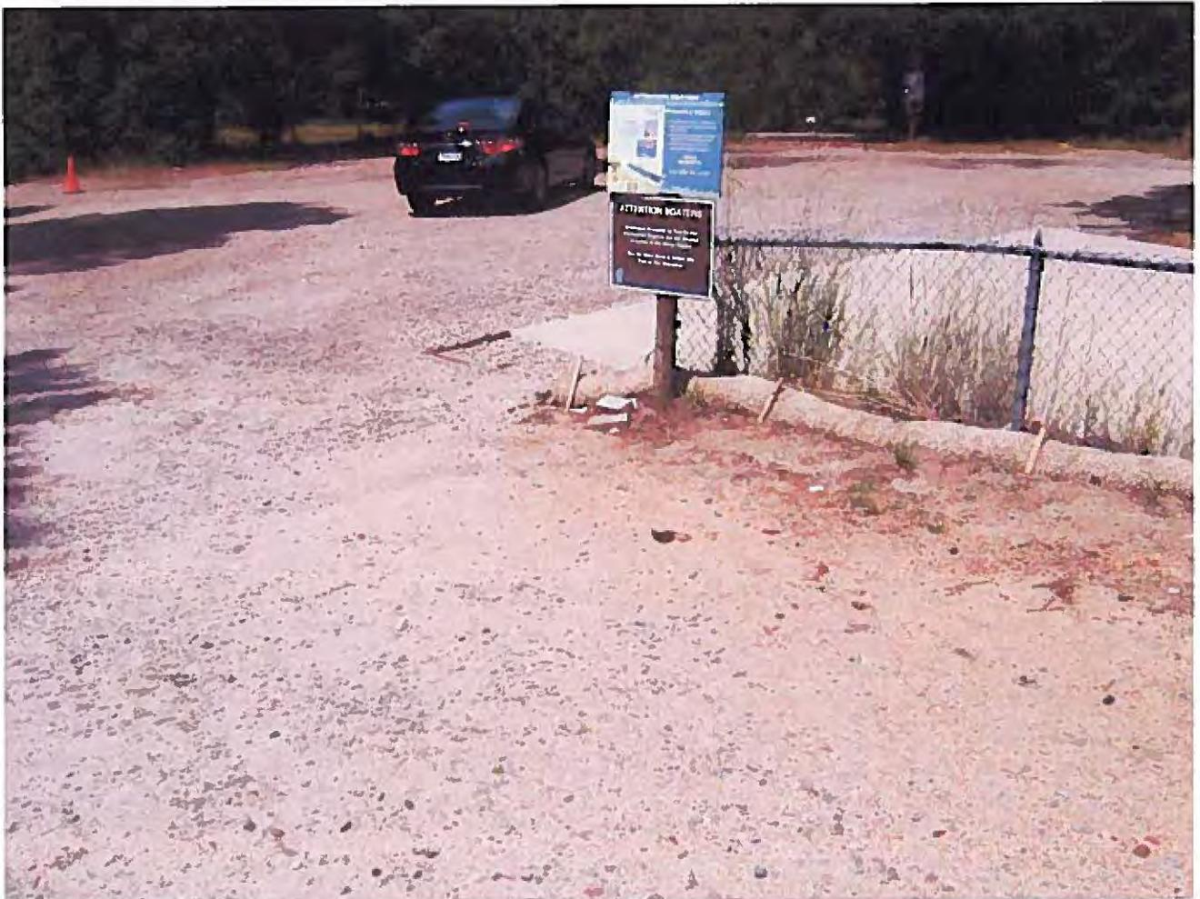
Photograph 04 - Looking East, Northeast at fiber roll. The fiber roll is not J-Hooked at its end which is also installed perpendicular to the grade lower than the rest of the fiber roll, and not parallel to the grade. Any runoff that flows toward the fiber will flow along it toward the downgradient end and, eventually, down the boat ramp and into the marina.
