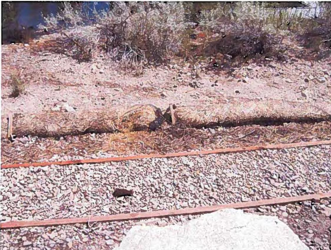
**Photograph 16 - Mid-way between 2nd and 3rd ramps west from the office. The fiber rolls have been slightly flattened, and the ends have not been overlapped leaving a gap between the rolls where stormwater runoff can become concentrated.**
