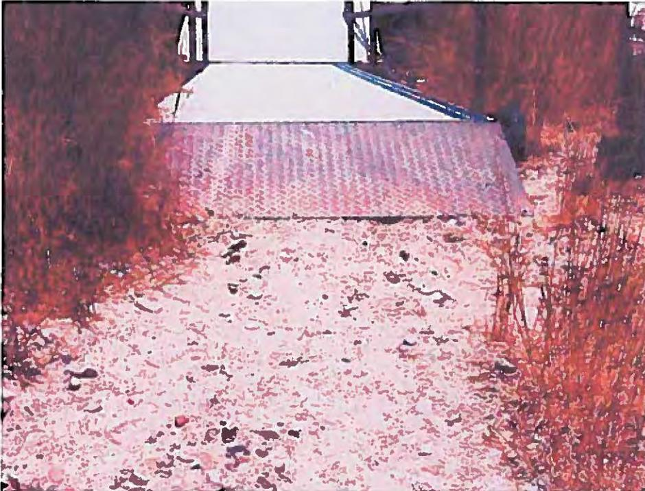
**Picture 2: The walkway is downward sloping from the parking lot to the gangways. Potential for rill or gully erosion into the marina surface waters is possible.**
