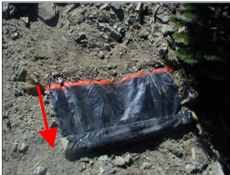
Figure 45. Erosion sediment fence to capture sediment from hillslopes, roadcuts, and culvert outlets. Red arrow indicates down slope direction.
