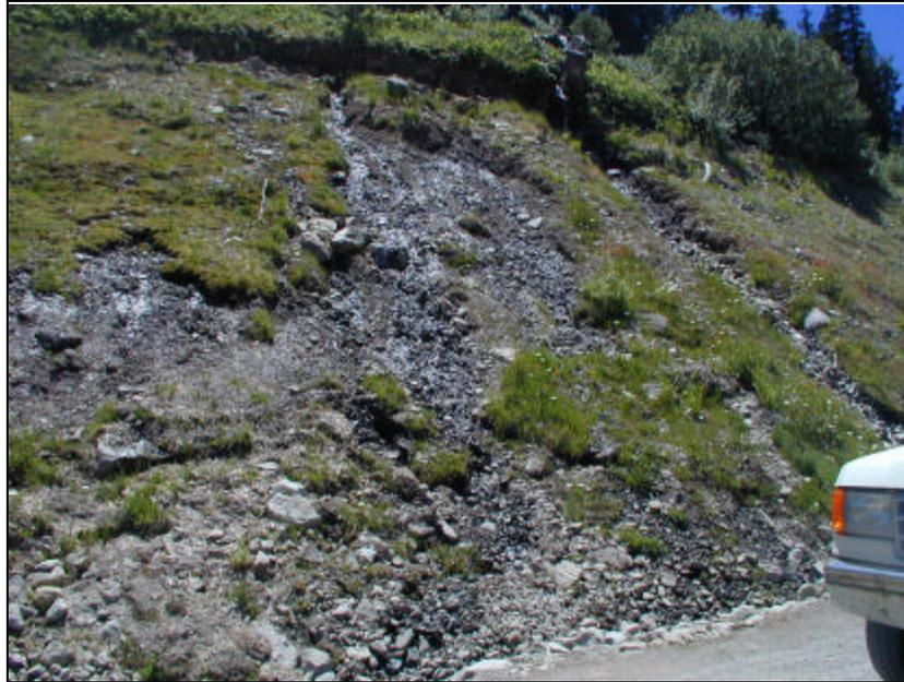
Figure 24. Interception of shallow groundwater on cutslope contributes to increased flow in ditches and road surfaces.
