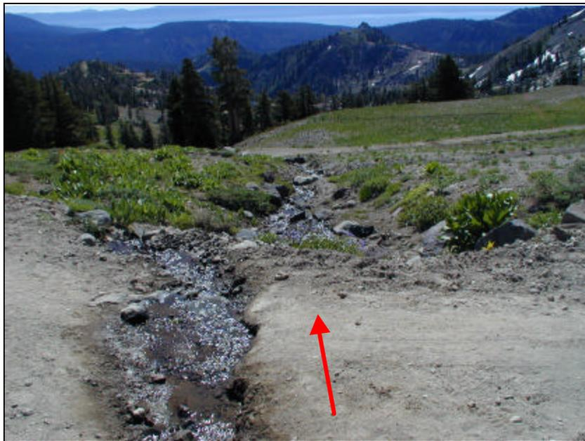
Figure 23. Gully formed on road surface concentrates and directs runoff and sediment to an adjacent stream channel in Sector IV. Red arrow indicates direction of flow.
