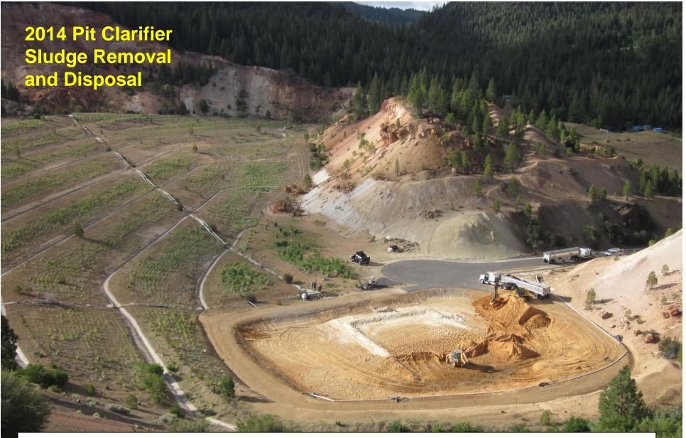
• Approximately 178 tons of sludge were hauled off site for disposal in July 2014.
