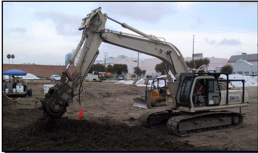
In-Situ Mixing of RegenOx™ On-Site
