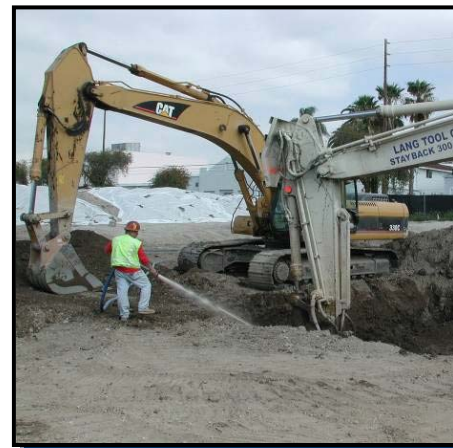
Soil Mixing and Excavation Activities
