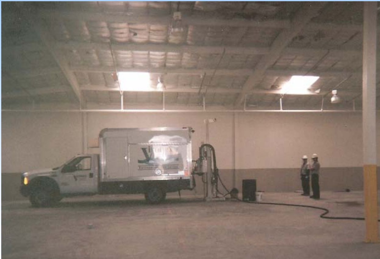
Direct Injection Through Pre-cut Holes in Concrete Floor
