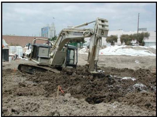
Treatment by the in-situ mixing application of RegenOx™
