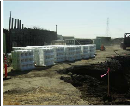
Figure 2. RegenOx Material On-site
