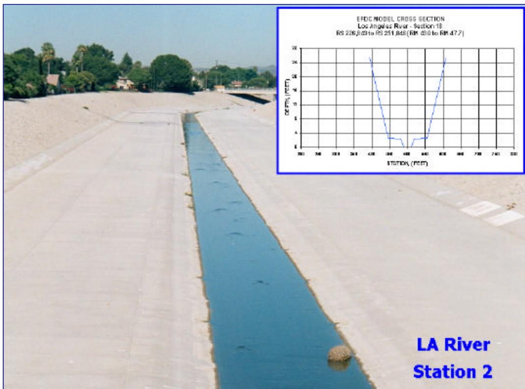
Figure 3-2a. Channel Cross-Section at LA River Station 2
