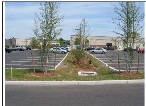
Figure 5-9. Typical Concave Bioretention System
