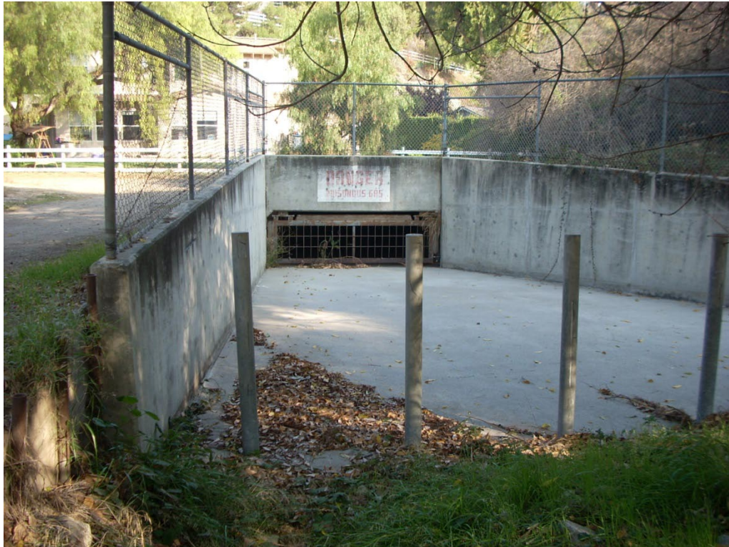
Figure 2.9 Chadwick Canyon Tier 2 Site Entering Subsurface Storm Drain
