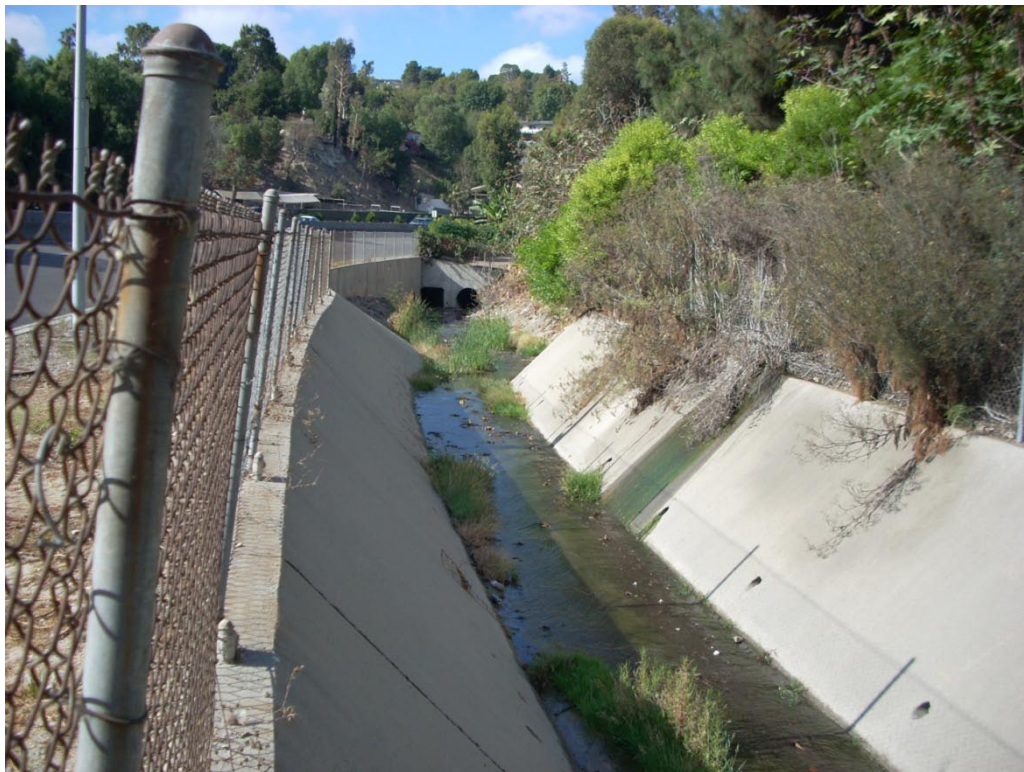
Figure 2.10 Looking South/Upstream RDD 275 along Crenshaw Boulevard
