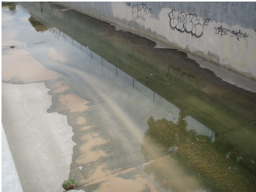
Figure A-4: Downstream of Site 3I_NORMP. Taken on March 1, 2011 at 11:30 a.m.
