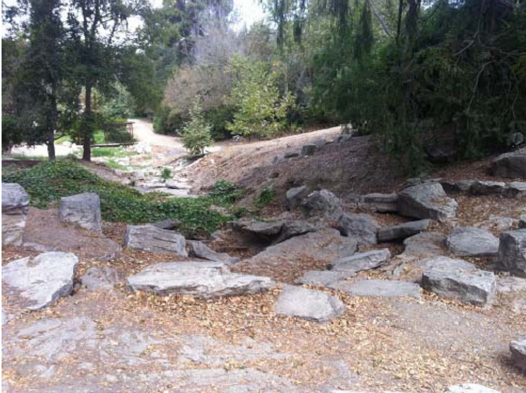
Figure A-7 - The South Coast Botanical Gardens Pond spillway, 20_SCBG, viewed from upstream looking downstream. Taken on September 28, 2010 at 1:15 p.m.
