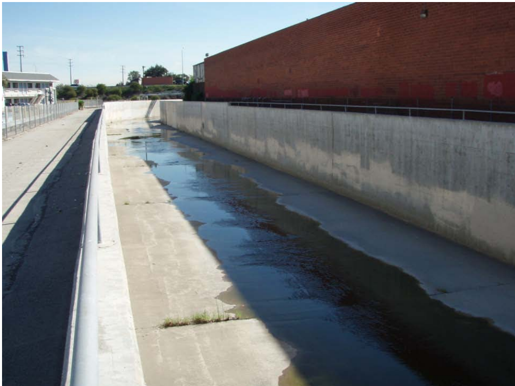
Figure A-6: Downstream of Site 30_VERSEP. Taken on November 4, 2010 at 12:00 p.m.
