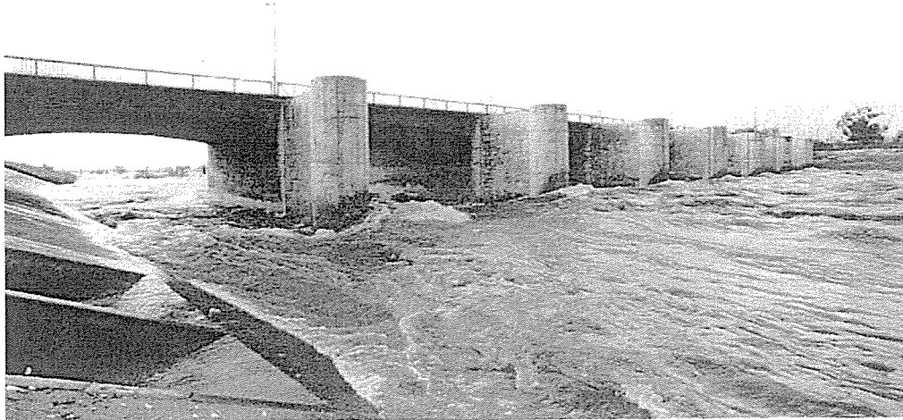
Willow Street Bridge Over the Los Angeles River
