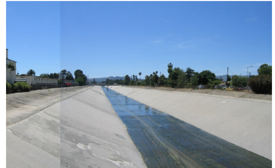
Existing conditions, trapezoidal section at Canoga Park. (2006)
