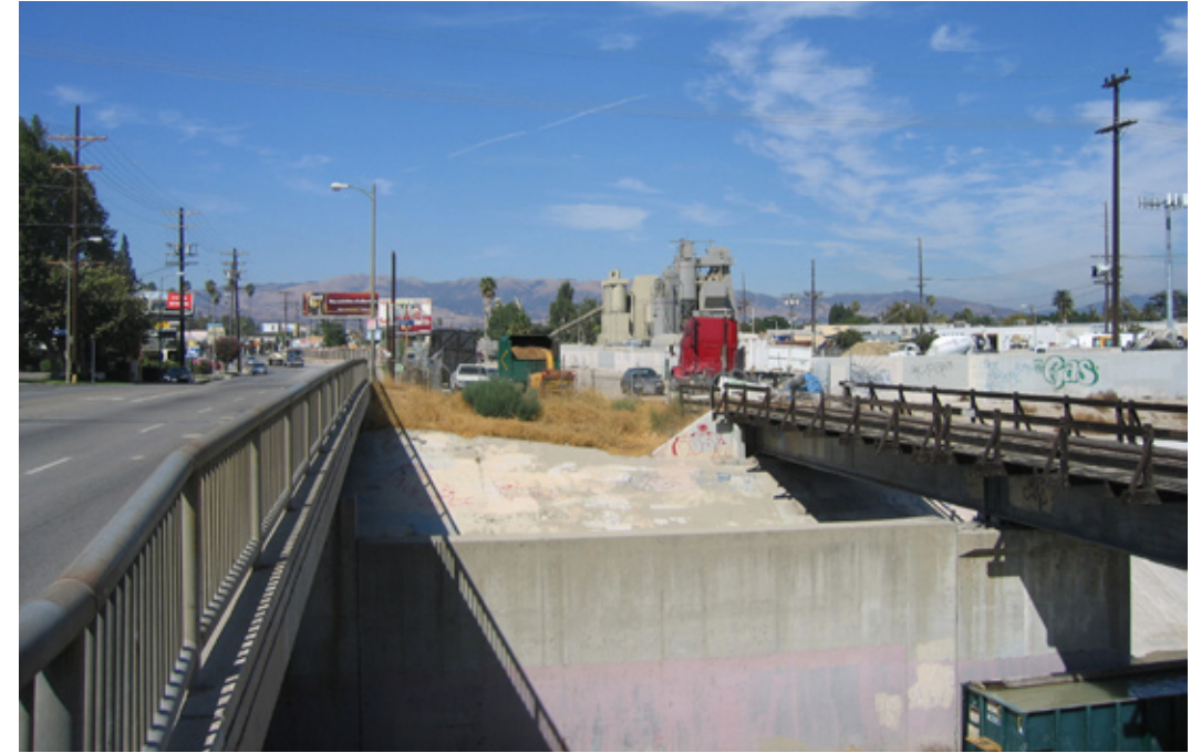
Existing - Looking north from the River's edge along the landscape material yards that front on Canoga Avenue in Canoga Park (2006)
