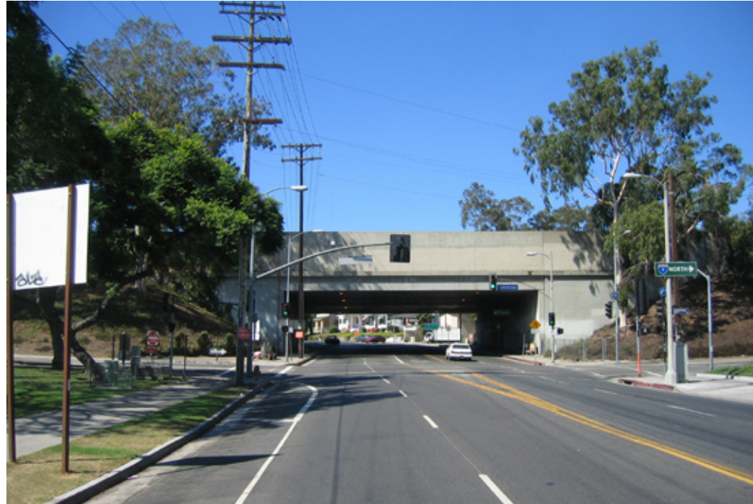
Existing - Looking west along Fourth Street at the Interstate 101 underpass towards Boyle Heights (2006)
