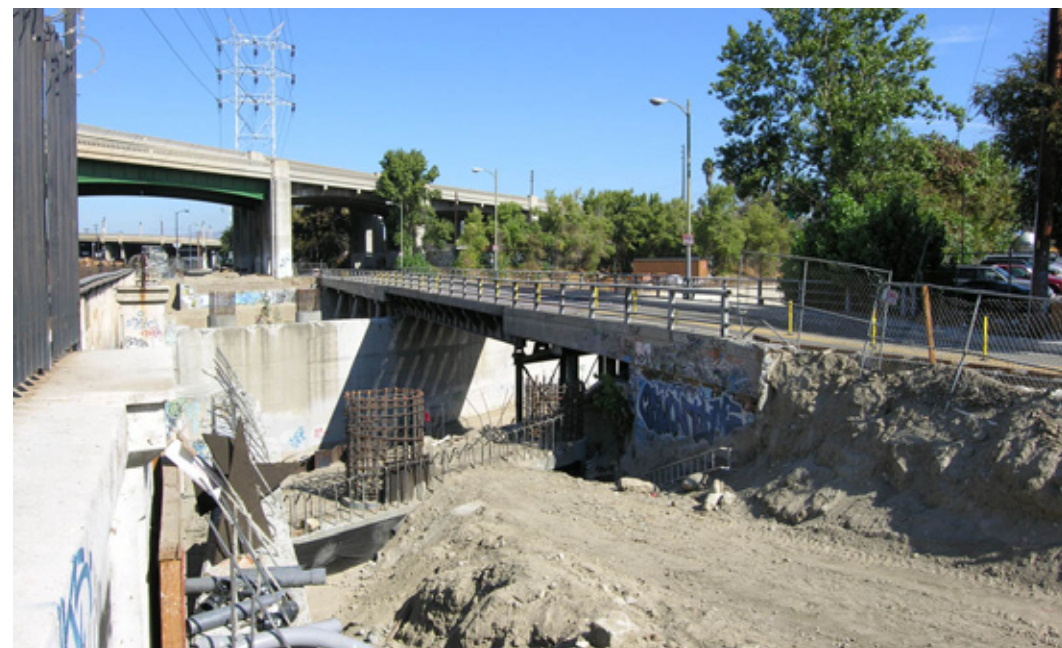
Existing - Avenue 19 bridge over the Arroyo Seco under construction (2006)
