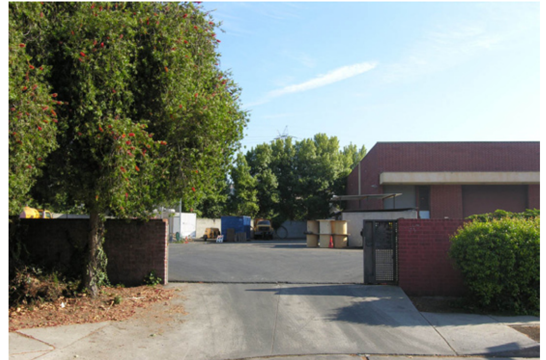
Existing - Termination of Dorris Place just north of the River (2006)
