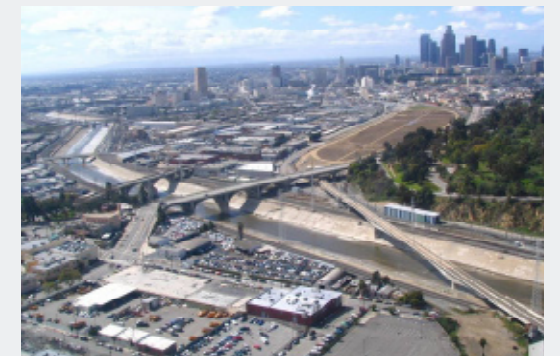
Reach 8: Taylor Yard to 1st Street (2006)
