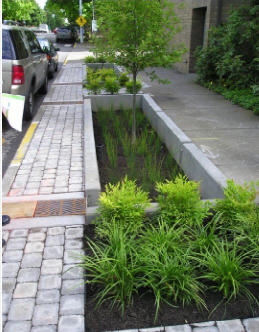
Bioinfiltration trenches treat runoff from adjacent roadways, and provide landscape amenities. (City of Portland, 2006)
