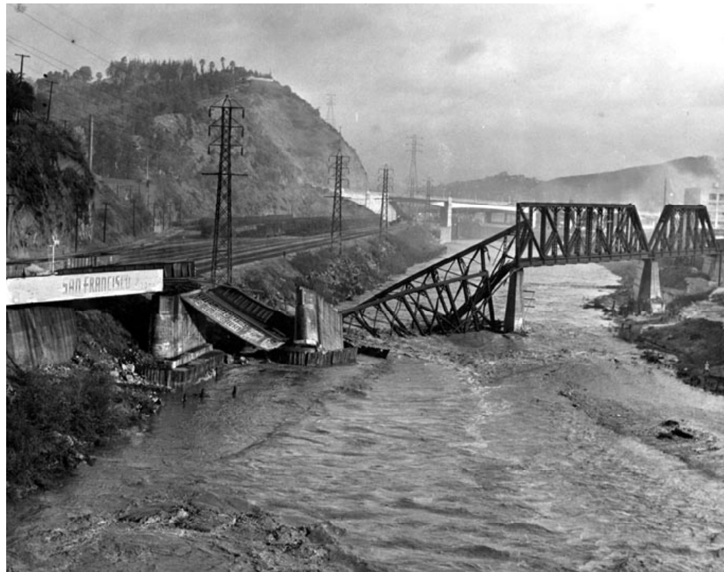
Flooding in 1941 washed out numerous bridges. (Los Angeles Public Library Photo Archives; used by permission.)
