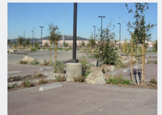
Porous pavement parking surfaces at the Río de Los Angeles State Park, provide detention and water quality treatment. (2006)
