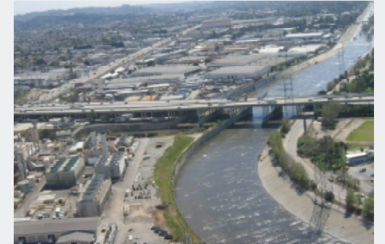
Reach 6: Burbank Western Channel to Taylor Yard (2006)
