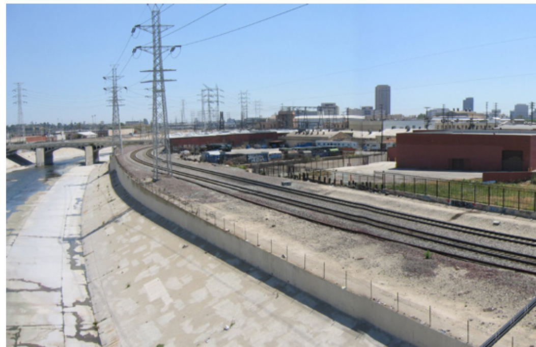
Existing rail lines separate the Department of Water and Power North Main Street facility from the River's edge. (2006)
