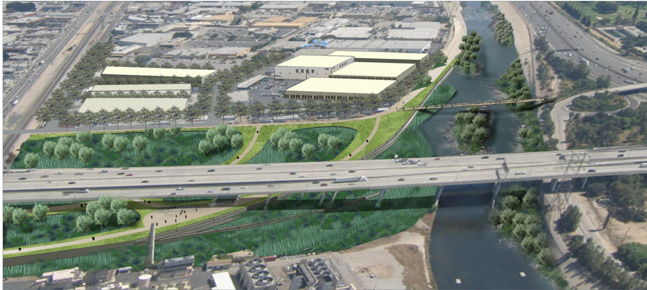
Water quality treatment at the confluence of Verdugo Wash and the Los Angeles River demonstrates a regional-scale approach to treatment.
