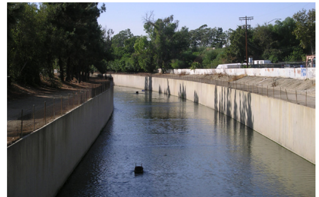
Existing conditions downstream of Sepulveda Dam to the confluence with Tujunga Wash. (2006)
