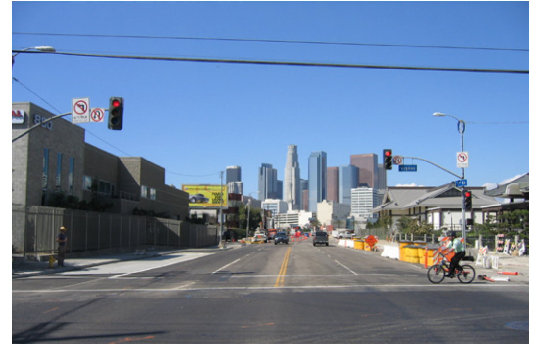
Existing - Looking west along First Street from the intersection of First and Vignes, with Downtown in the distance and construction of the Gold Line East Side Extension on the right. (2006)
