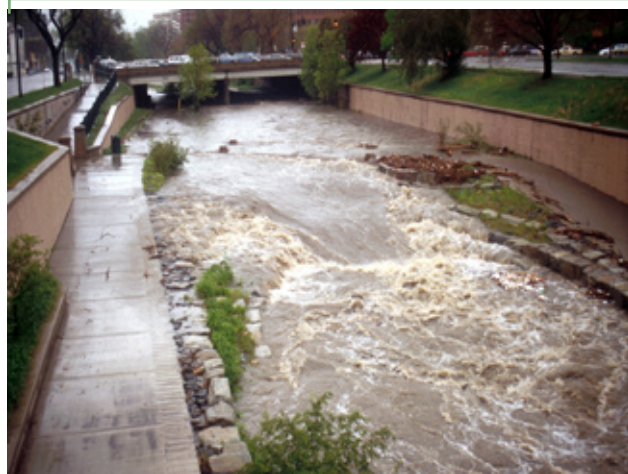
Flooding along the Cherry Creek in Denver, Colorado (2006)
