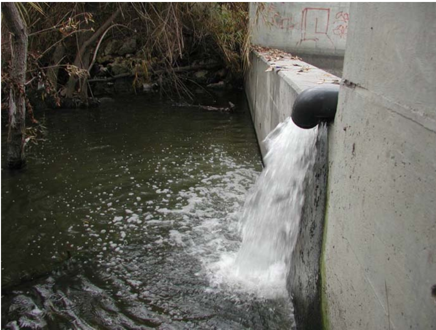
Figure 6. Energy dissipater end wall and Discharge Point for Treatment System Effluent
