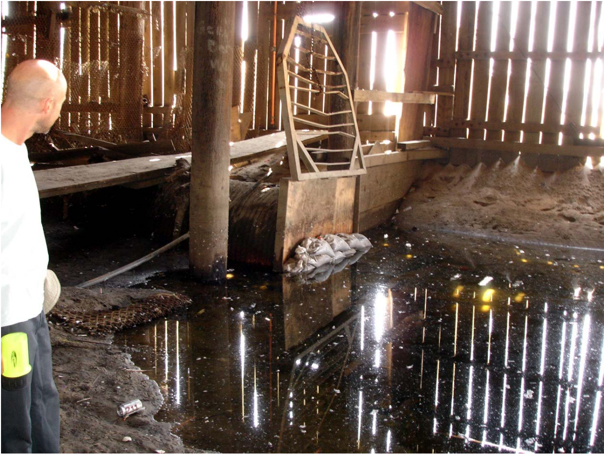
Photo 1: Storm Drain Diversion
