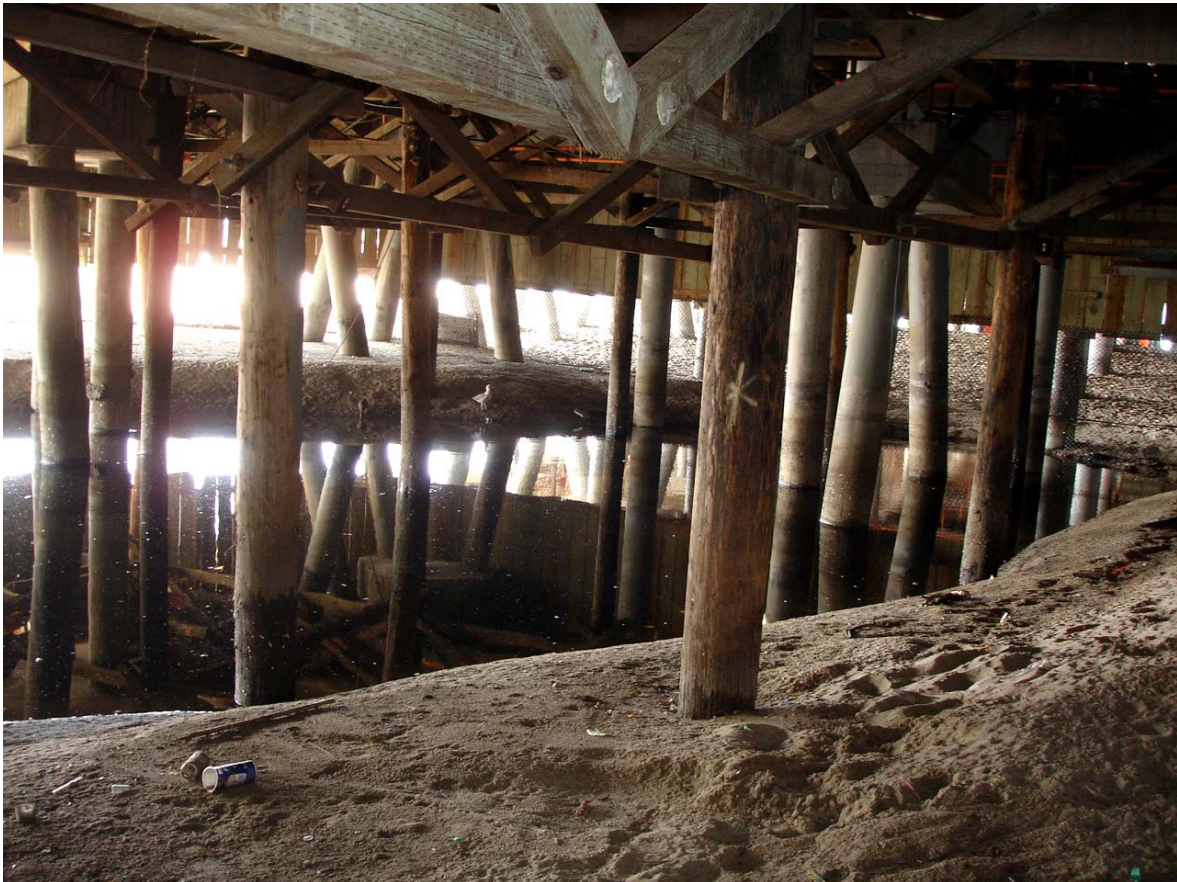
Photo 4: Poned area west end
