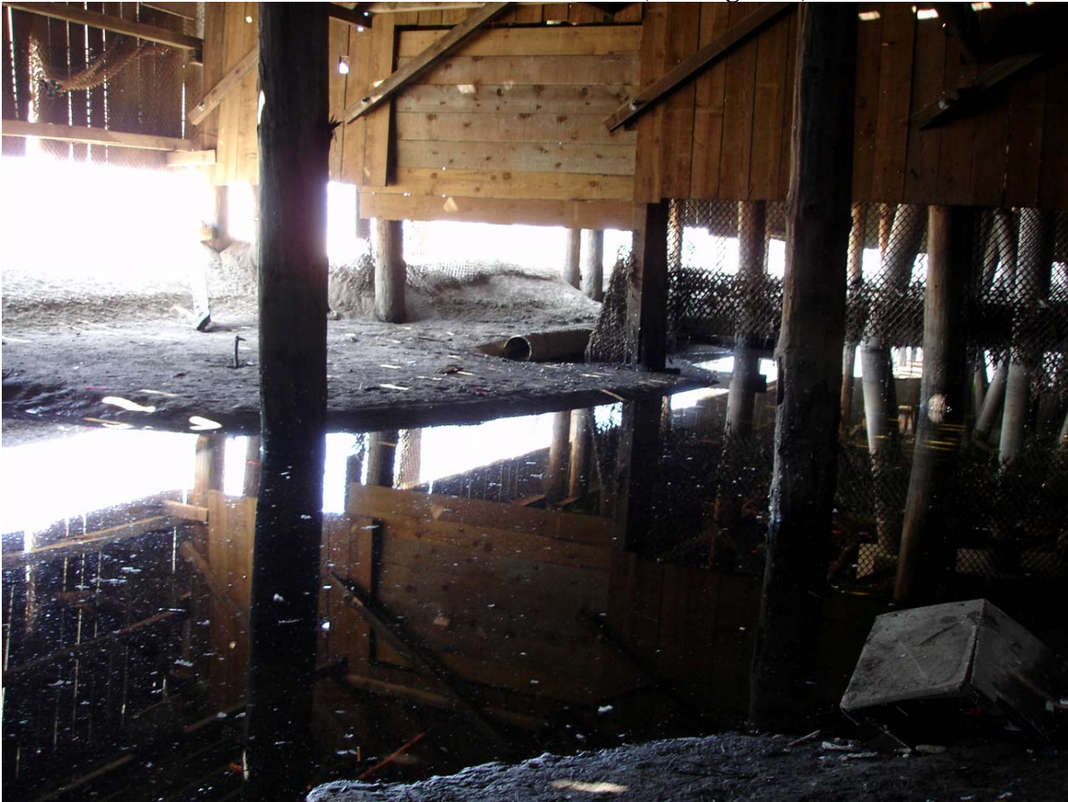
Photo 3: Poned area east end (looking west)
