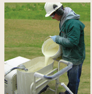
FIGURE 1: FILLING A PUMP WITH ORC ADVANCED SLURRY
