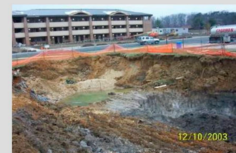
Figure 5. Former Tank Basin Excavation
