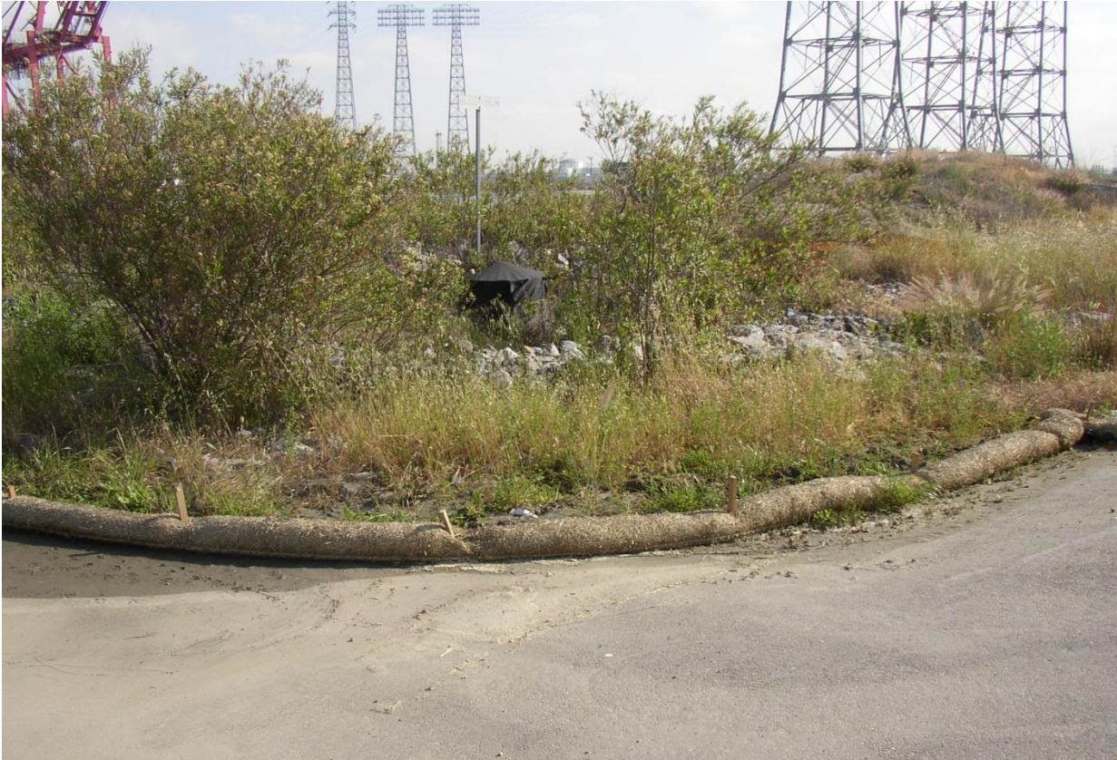
Photo 2 – Unpaved and Vegetated Area
