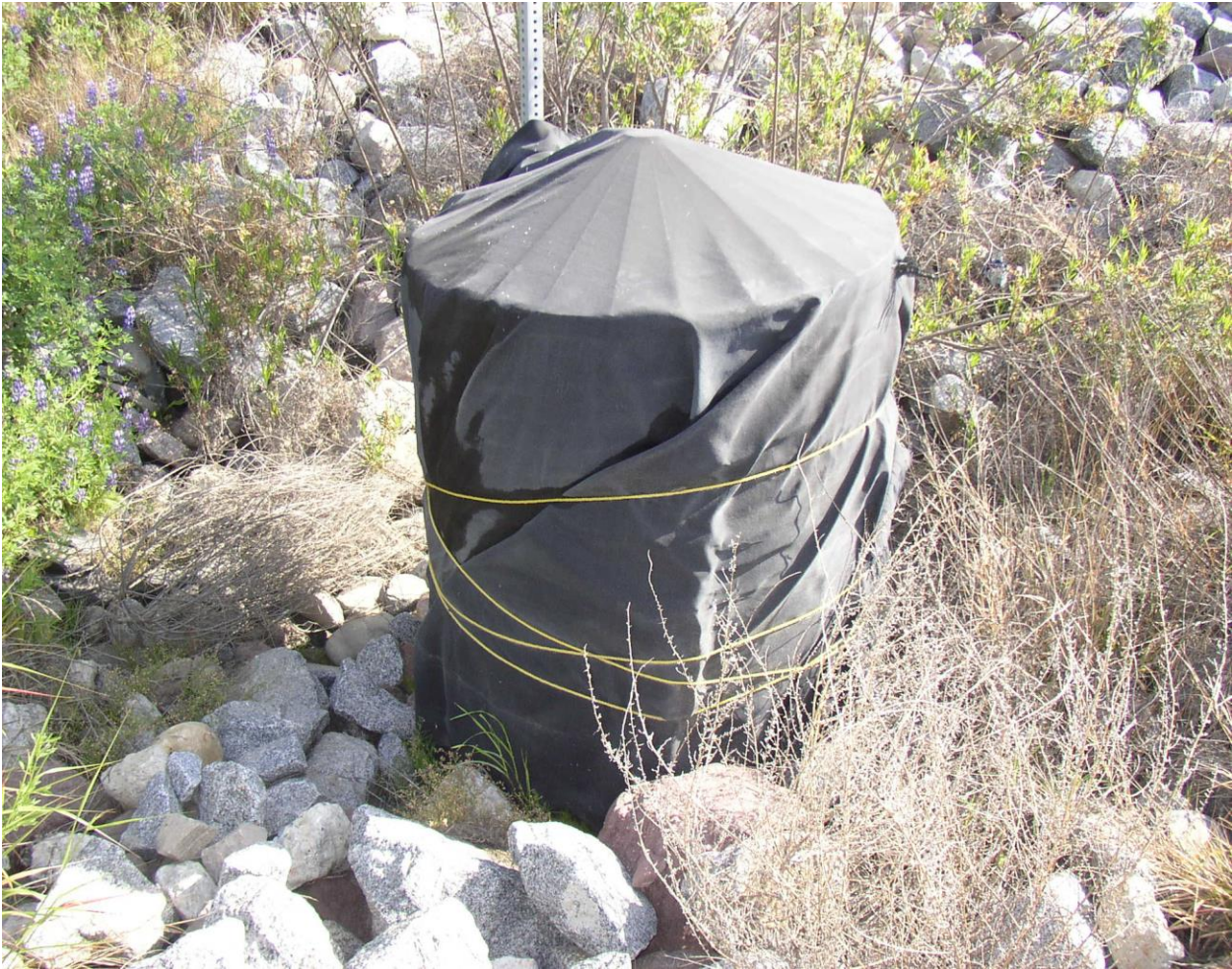
Photo 3 – Riser Wrapped in Filter Fabric
