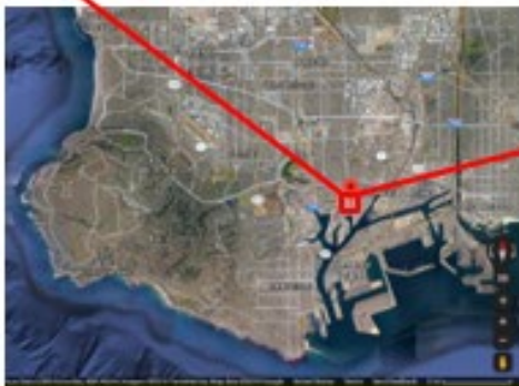
The Marine Tank Farm Divided with Areas A, B, and C (Before Property Demolished and Converted)
