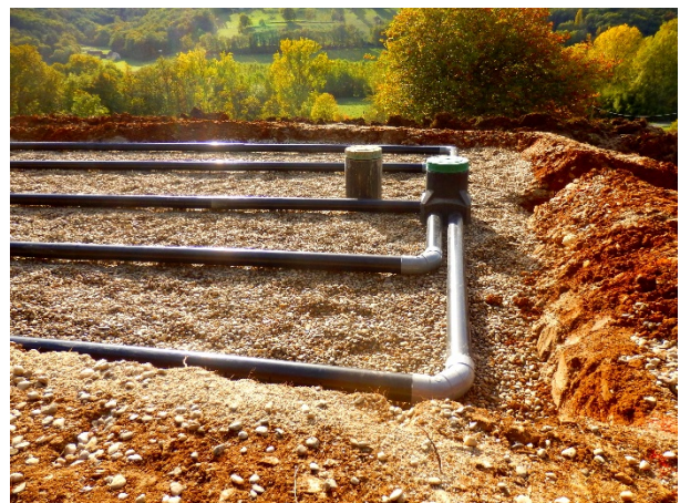
Construction of a Leach Bed
