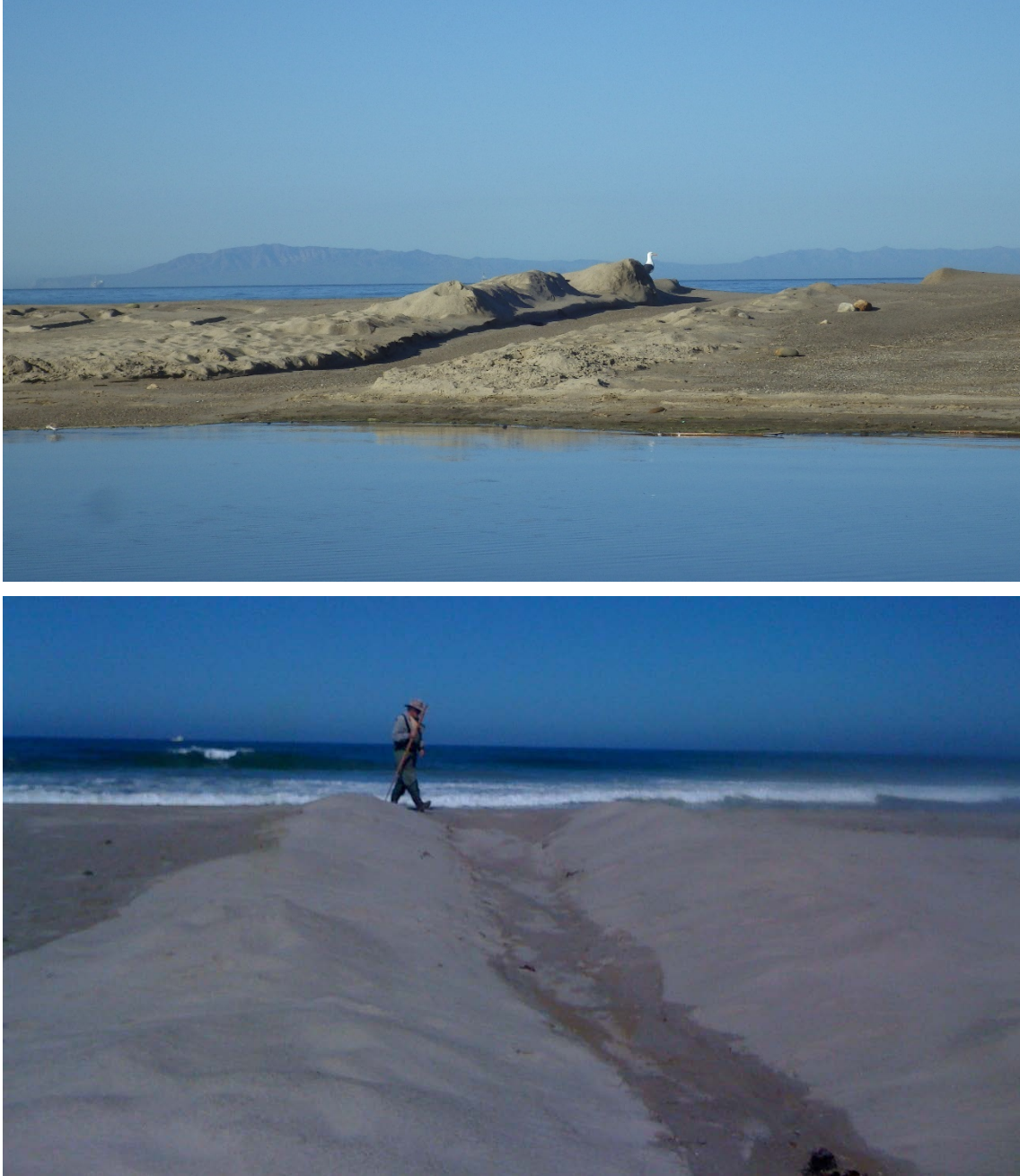
Figure 3-25. Photographic examples of a manually dug trench through the north end of the SCRE beach berm taken on March 21, 2016 (top) and July 20, 2016 (bottom). [Source photographs from ABC Laboratories.]
