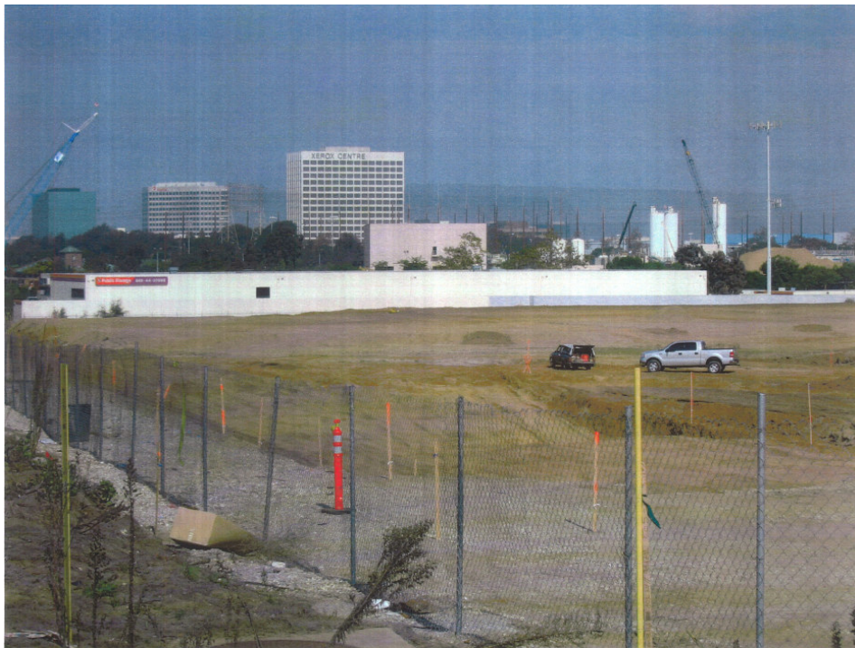
2005: Post grading and before new building construction
