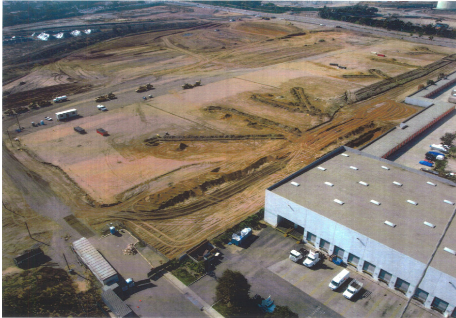
2005: Deep soil vapor remediation system installation
