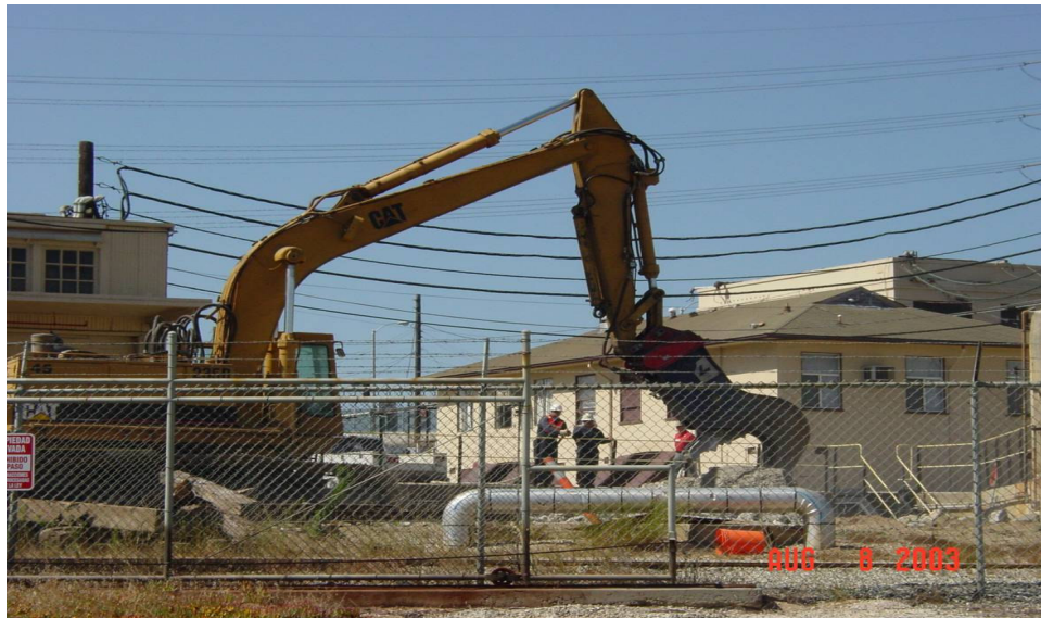
August 2003: Site demolition in progress
