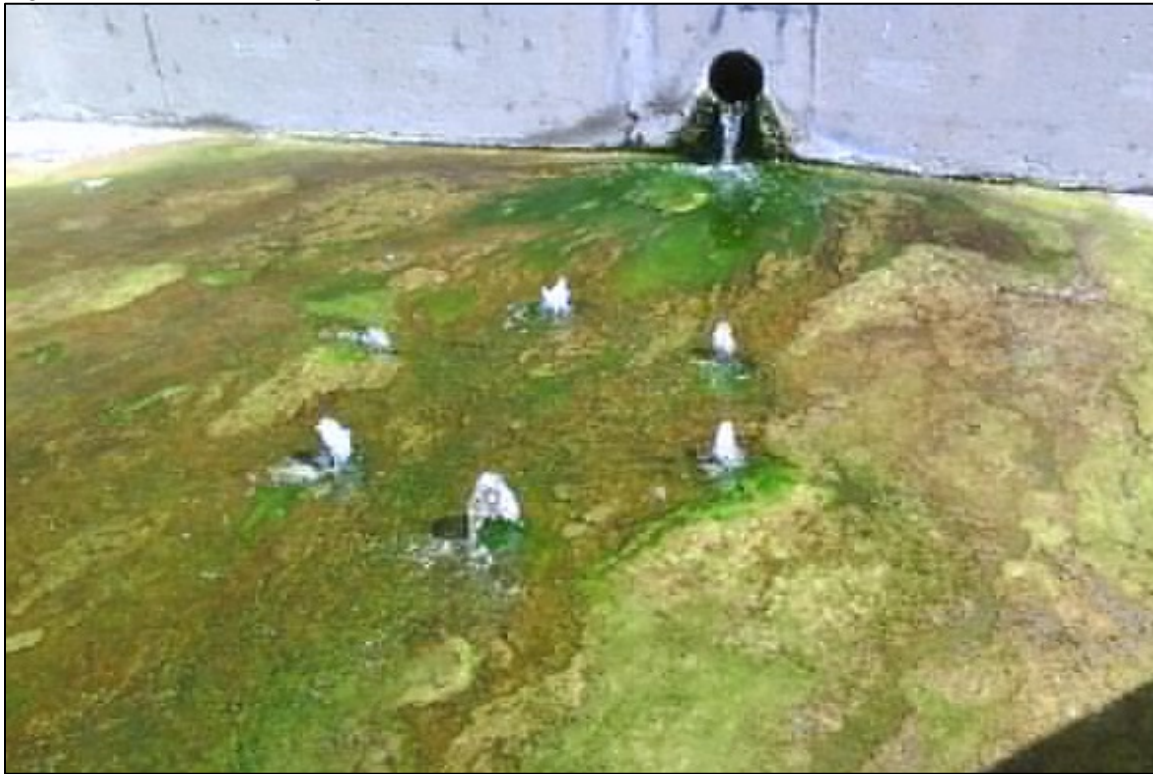
Figure 2. Manhole Exuding Groundwater into San Jose Creek
