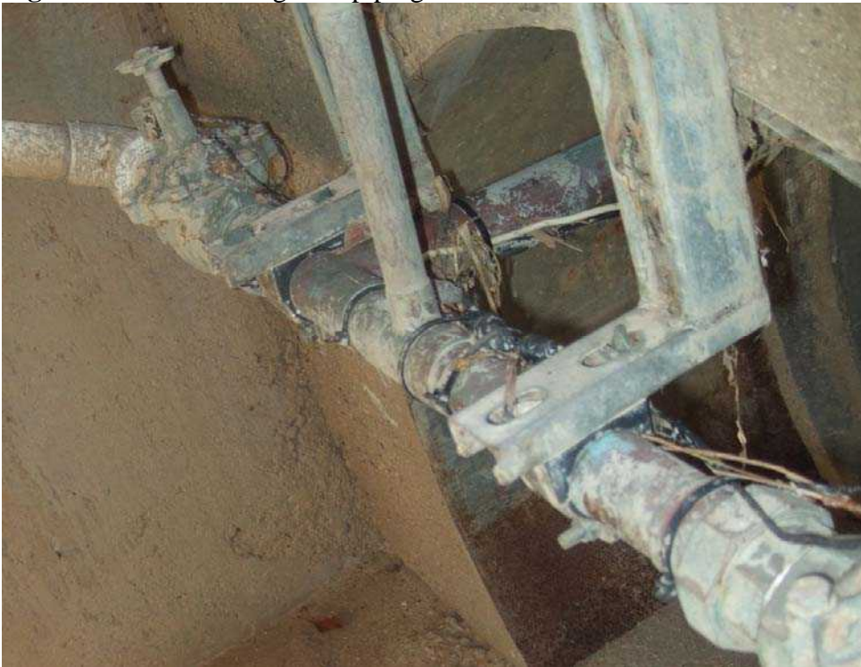
Figure 2-4. Private irrigation piping in storm drain
