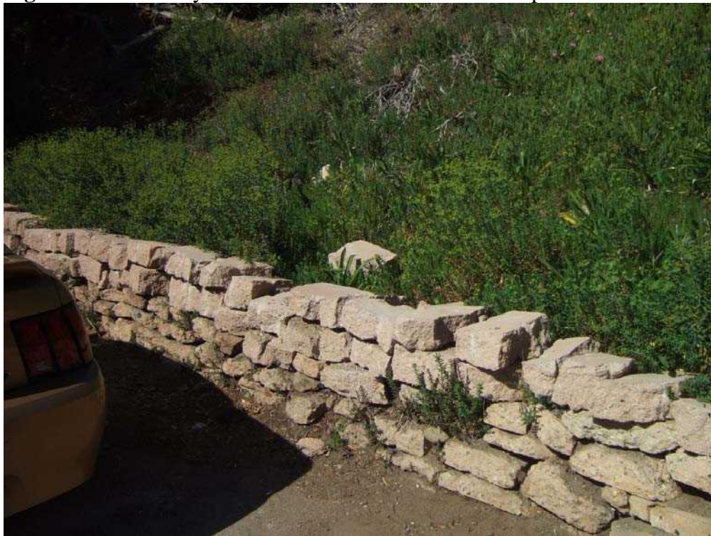
Figure 2-7. Privately constructed waste concrete hardscape
