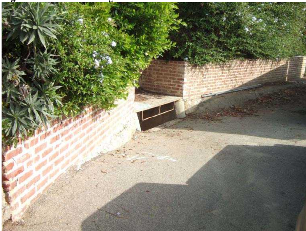
Figure 2-8. Brick retaining wall
