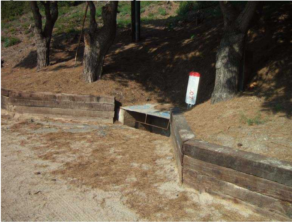
Figure 2-9. Treated wood retaining wall
