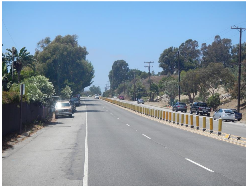
Figure 7-14. Pacific Coast Highway Near Escondido Beach
