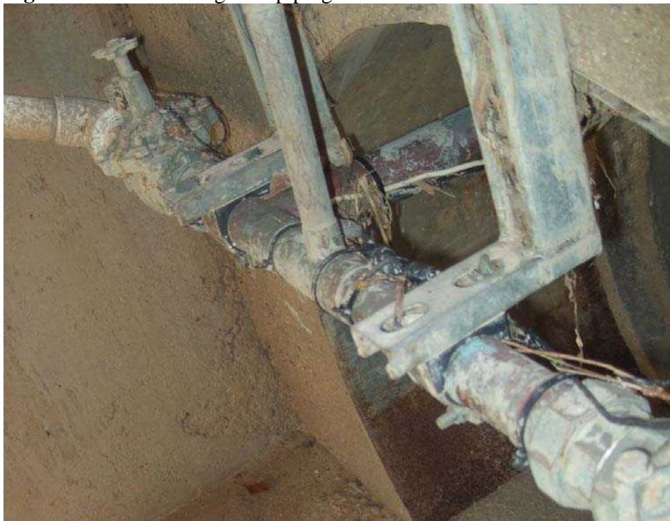
Figure 2-4. Private irrigation piping in storm drain
