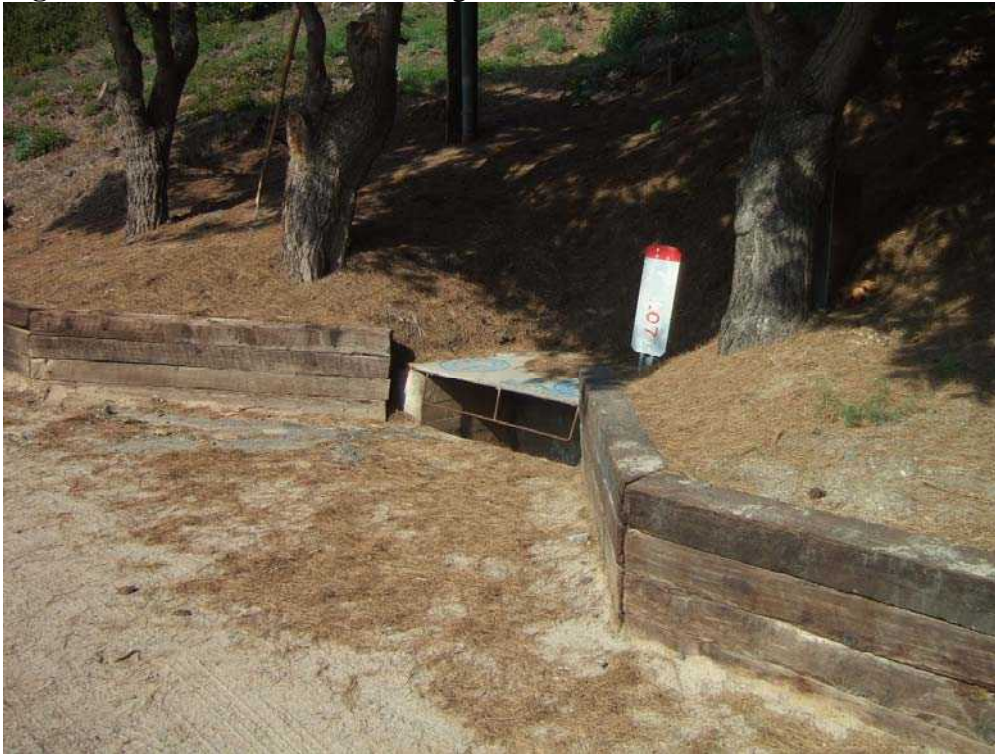
Figure 2-9. Treated wood retaining wall
