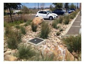
Figure 5-11 Recently Constructed Biofiltration in a Parking Lot
