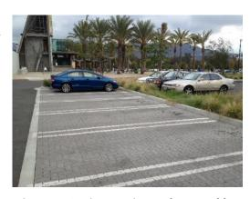
Figure 5-10 Bioretention and Permeable Pavement at the Los Angeles Zoological Park
