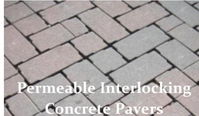
Permeable Interlocking Concrete Pavers
