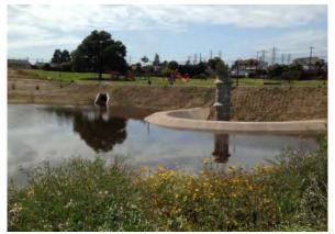
Basin was modeled as an infiltration basin. The basin includes a small permanent pool (1500 cubic feet), the volume of which was excluded from the calculation of total storage capacity.
