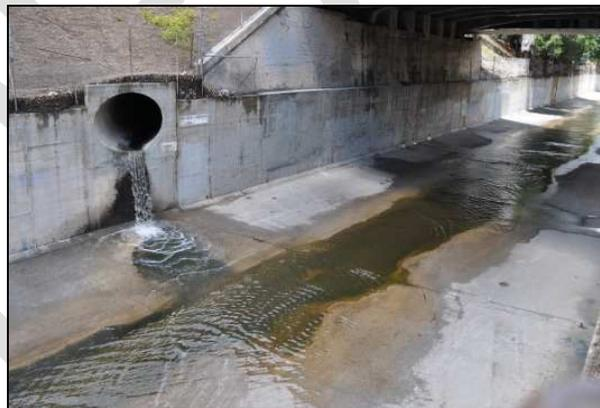
The field screening points are representative of discharges from the City which are a mix of residential and commercial land uses. Stormwater discharges from the outfall field screening points will be measured against ambient TMDL standards. The ambient standard is
