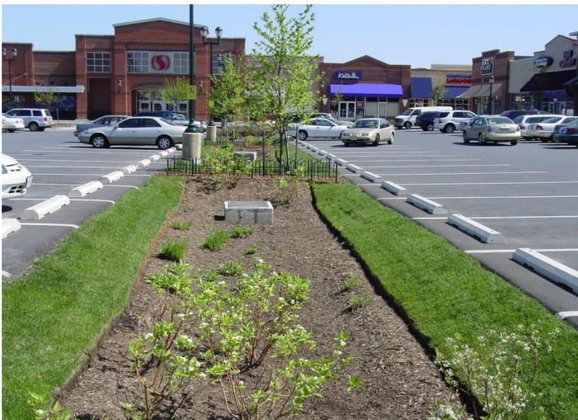
Figure 13: Bioretention BMP
