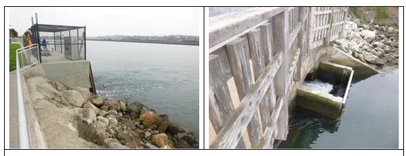
Figure B-2. Tide Gate Separating the Grand Canal from MdR Harbor (Ebbing Tidal Conditions)
