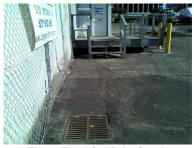
Figure 14. Example Catch Basin at Seamark
