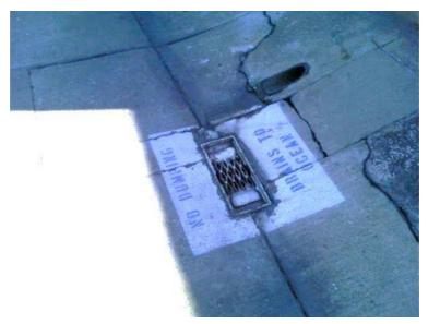
Figure 5. Windward Catch Basin Stenciling
