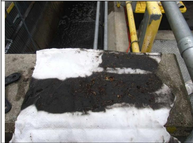
This is a typical filter from a to moderate size storm, but without sufficient intensity to fully submerge the filter. Without full submergence, sediment only accumulated along the bottom of the filter where there was a flow.
