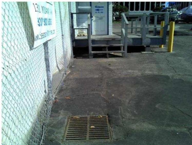
Figure 14. Example Catch Basin at Seamark
