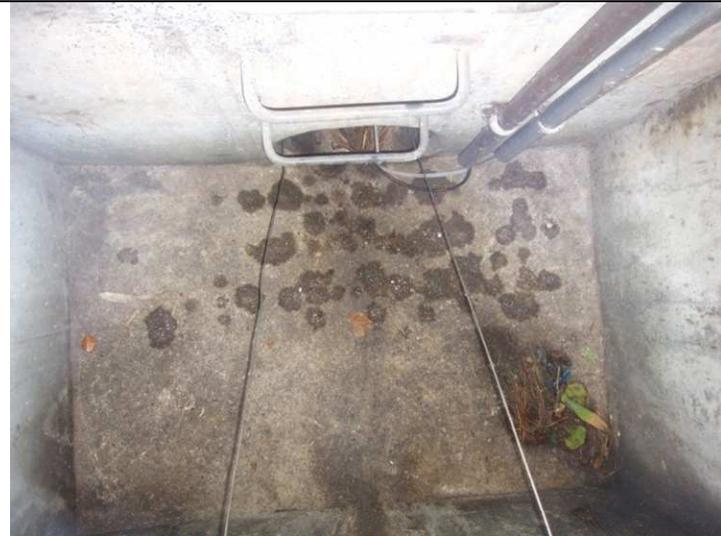
For retrieval the device is retrieved using the tethers to pull the device out of the catch basin lateral. In six events the device was removed without issue or need to enter the catch basin for retrieval.
