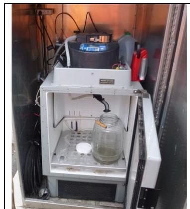
**Figure B-3. ISSCO Type Automated Flow and Sampling Equipment**
