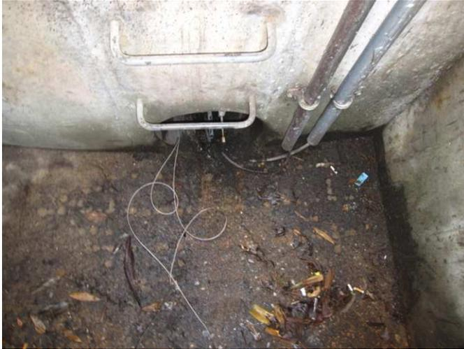
The deployment of the sample device involves pushing it into the catch basin lateral beyond the existing stormwater sampling equipment to reduce the chance of the sampling device snagging on the installed equipment.
