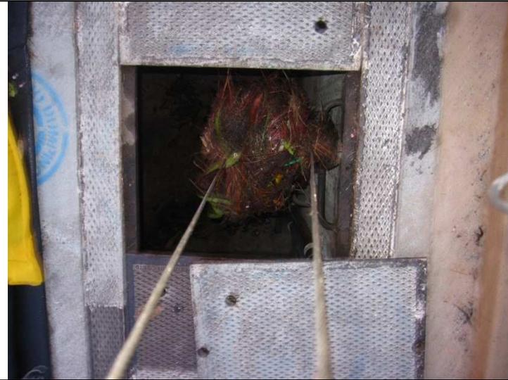
Excessive buildup of leafy debris occurred during one event, however since the catch basin was not entered some of this debris may have snagged on the device during removal.
