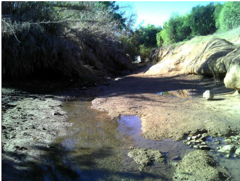
ESGV_LOW_DS Looking Downstream
