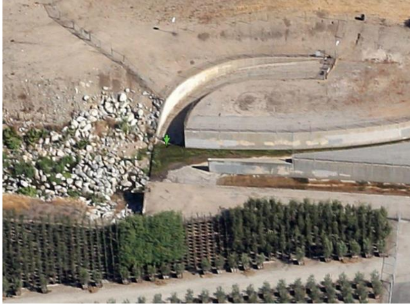
ESGV_LOW_DS Marshall Creek Flow Monitoring Location Aerial View
