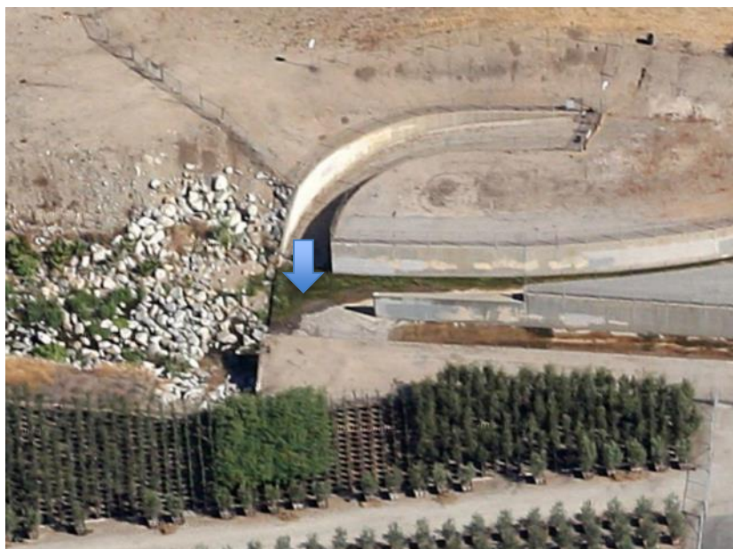
Figure 2-4. Confluence of Channels Discharging to Puddingstone Reservoir at Transition Between Hard and Soft Bottom Channel.
