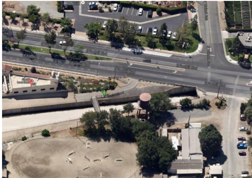
MTD 766 Aerial View
