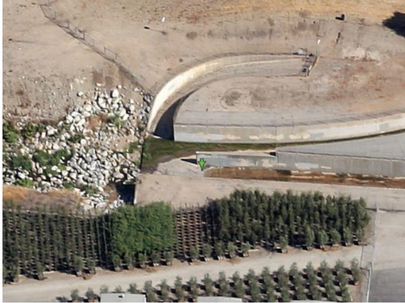
ESGV_LOW_DS Live Oak Wash Flow Monitoring Location Aerial View
