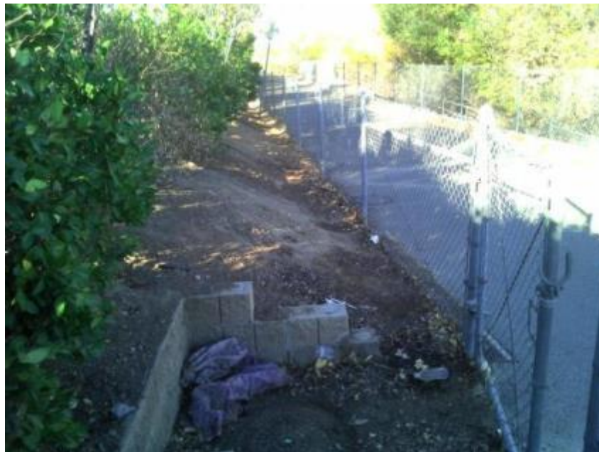
MTD 1510 Ground-Level View
