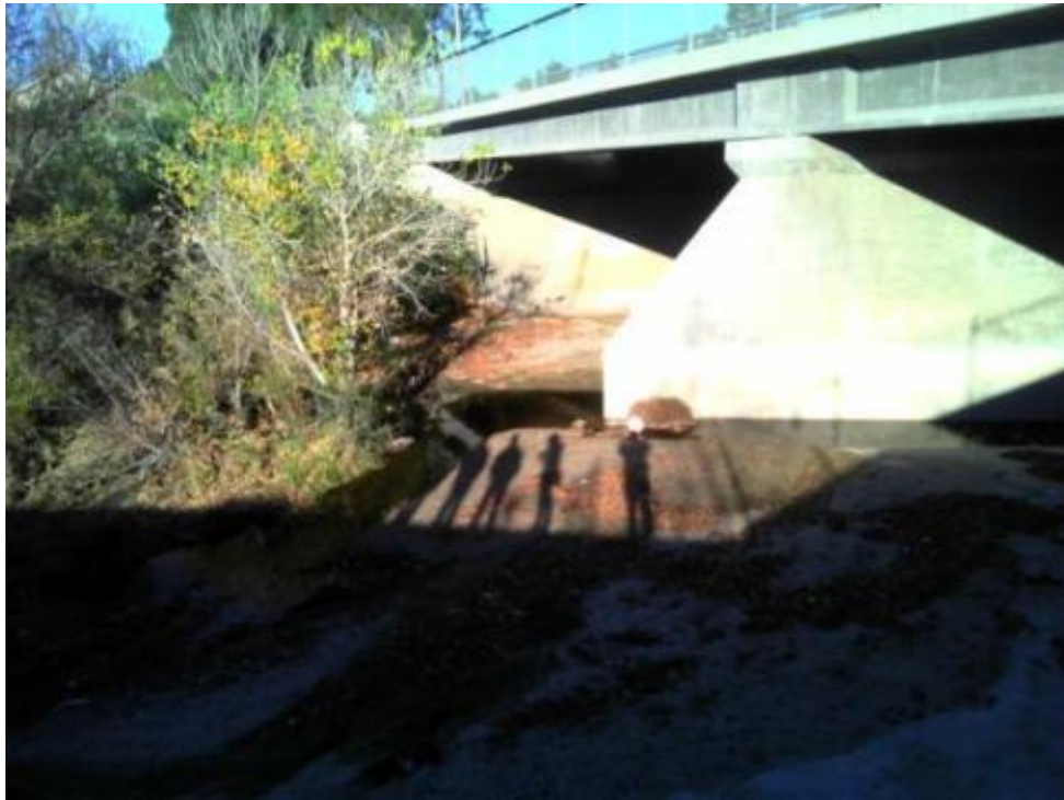
SNTCLR_BC_SWAMP Ground-Level View
