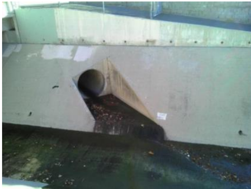
PD 1256/PD 1713 Ground-Level View
