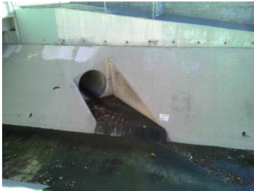
PD 1256/PD 1713 Ground-Level View
