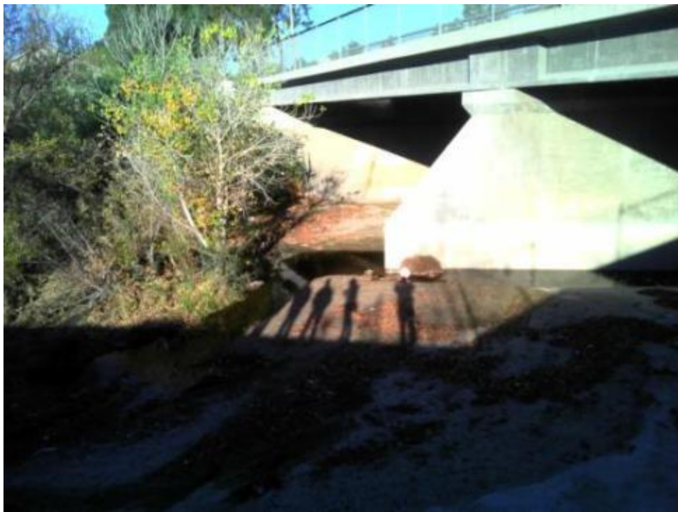
SNTCLR_BC_SWAMP Ground-Level View
