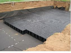
Figure 5-5. Subsurface infiltration gallery being constructed below a public park (source: Tetra Tech)
