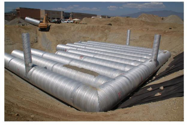
Figure 4 Photograph Storage/Detention System Using CMP (Contech, 2015)
