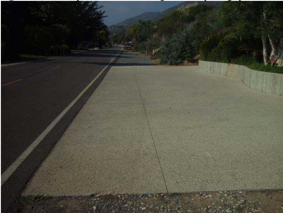
Figure 2-6. Cast in place concrete retaining wall with parking apron
