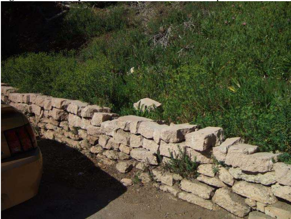
Figure 2-7. Privately constructed waste concrete hardscape
