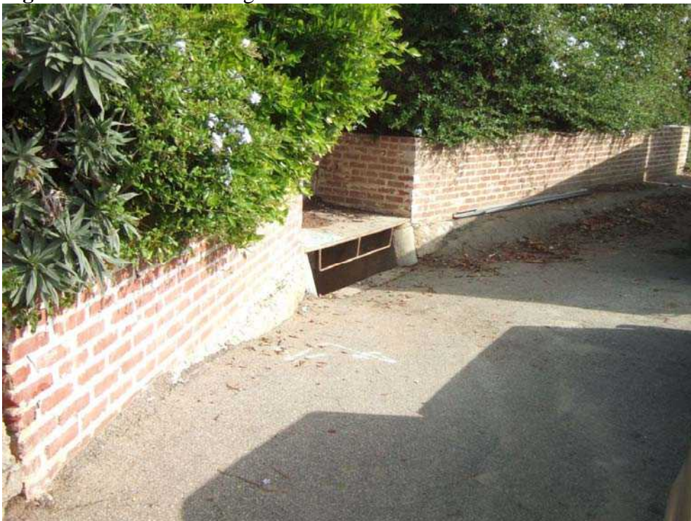
Figure 2-8. Brick retaining wall
