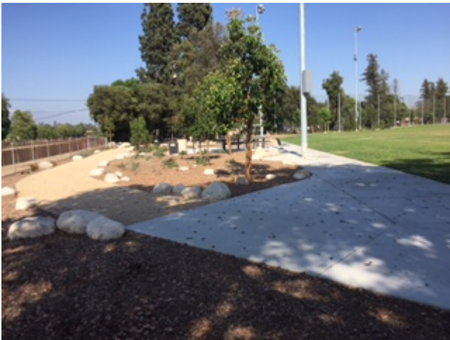
Infiltration trench and dry wells
