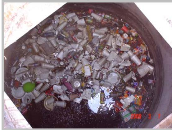
**Figure 3.4 Typical CDS unit contents after storm event**
