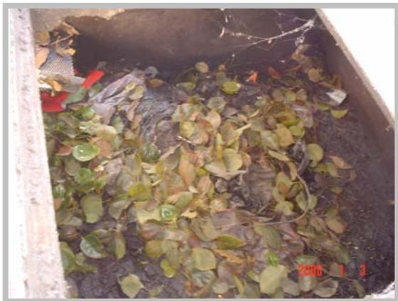
**Figure 3.2 Typical CB insert with vegetation in catchment area**
