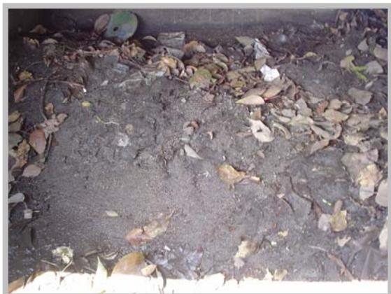
**Figure 3.3 Typical CB insert with sediment in catchment area**
