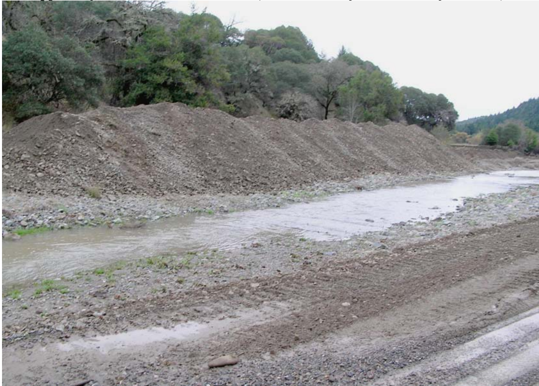
Photo 4. Stockpiled sediment and gravel from unauthorized construction of a new active wetted channel in Upper Dry Creek. December 2005 (Photo taken by Corrine Gray of DFG).
