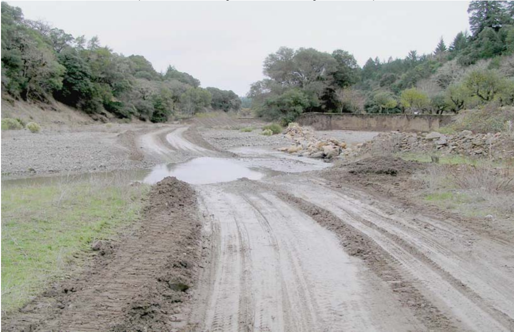
Photo 4. Stockpiled sediment and gravel from unauthorized construction of a new active wetted channel in Upper Dry Creek. December 2005 (Photo taken by Corrine Gray of DFG).
