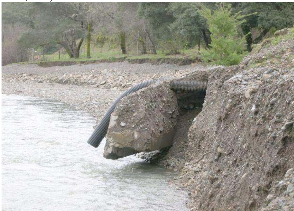
Photo 4. View facing downstream towards K-rail buried in the streambank. (Photo by Karen Maurer, March 6, 2006)
