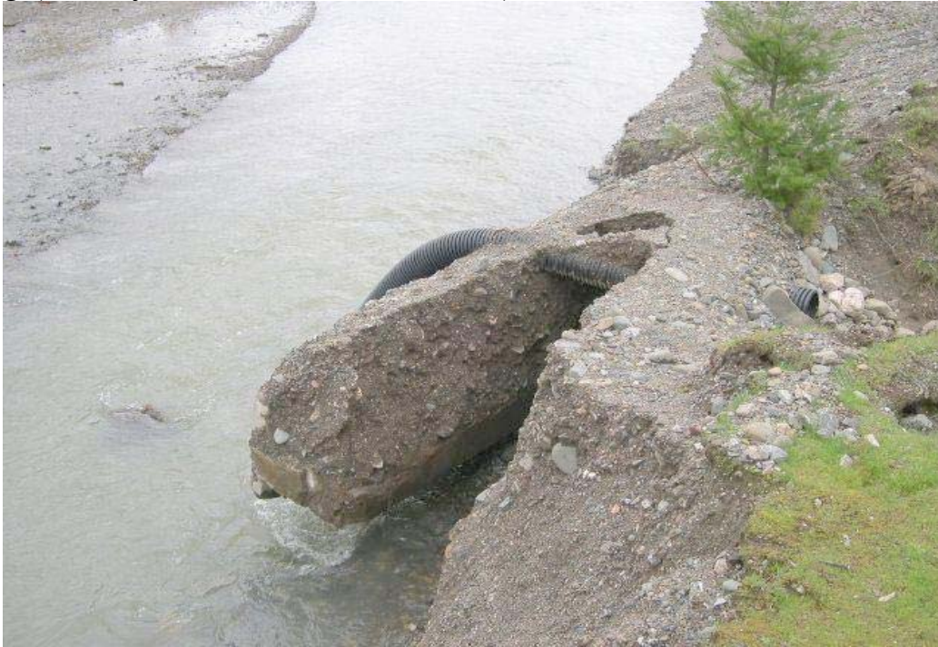
Photo 3. Overview of concrete K-rail buried in the streambank, with active erosion of gravels occurring. (Photo by Karen Maurer, March 6, 2006)
