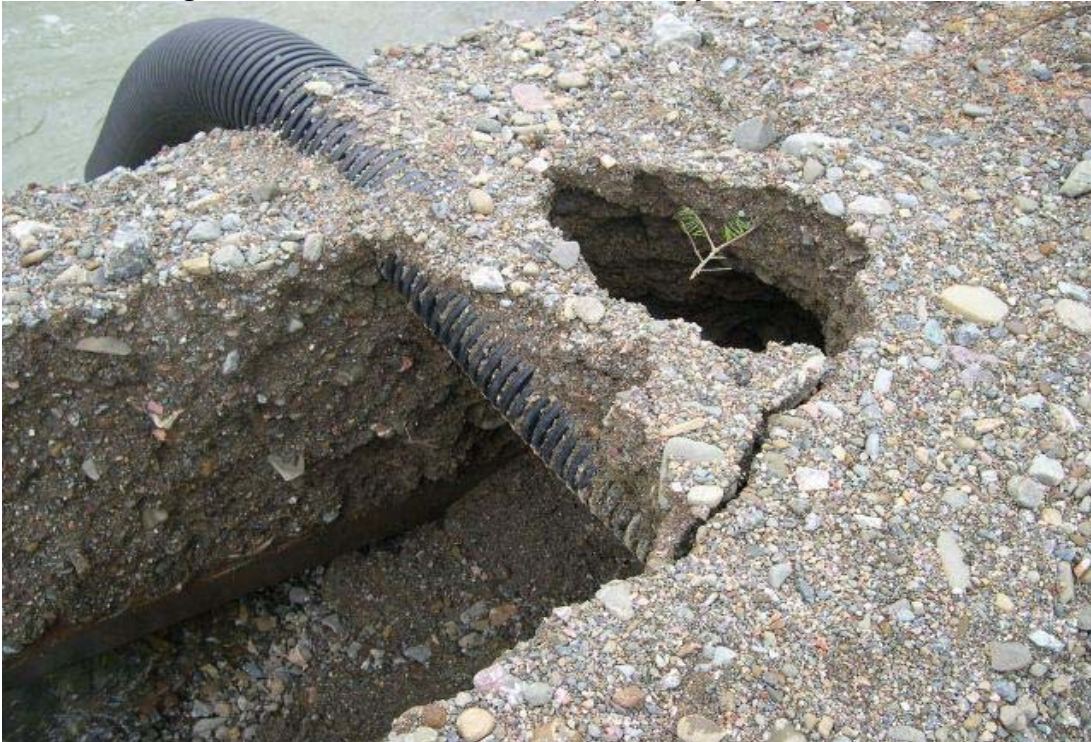
Photo 2. Erosion of gravels behind concrete K-rail. (Photo by Karen Maurer, March 6, 2006)
