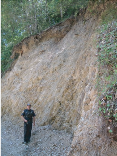
Loose sidecast on ~90% slopes into creek generated from excavation at top of driveway.
