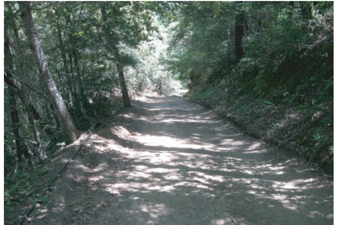
Midslope portion of undrained driveway that contains an outside berm.
