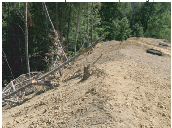
Debris exposed in fill slope along pad 1.
