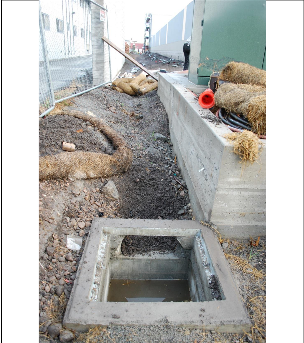
Photo 11: Southwestern drop inlet containing residual storm water with a pH of 9.65 and an undisturbed turbidity of 171 NTU.
