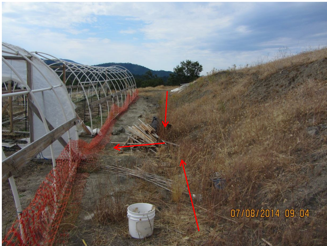
Image 16 – The arrows denote the constructed ditch drainage behind the four small greenhouses; the drainage is designed to carry all flows to the center of the greenhouses where it is then directed to the Class II stream below. This design concentrates flows, and may concentrate nutrients from the grow site potentially delivering these nutrients to the stream down slope. (Photo 6986)
