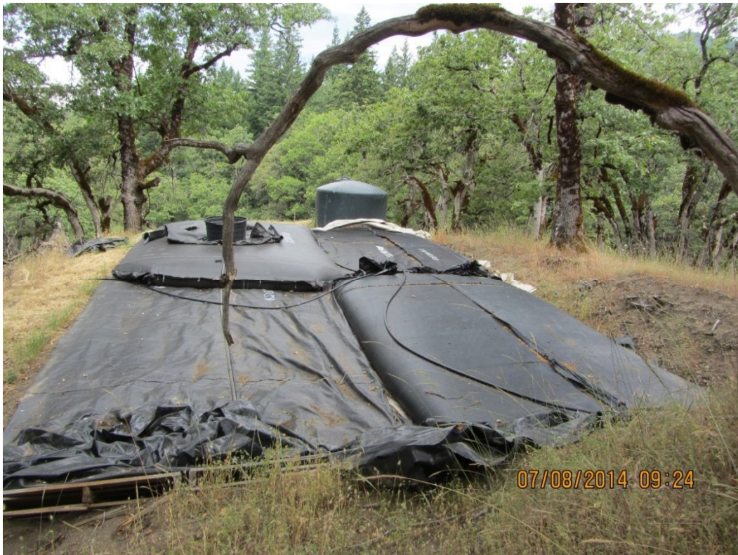
Image 7 – Water bladders and water tank (Photo 6998)
