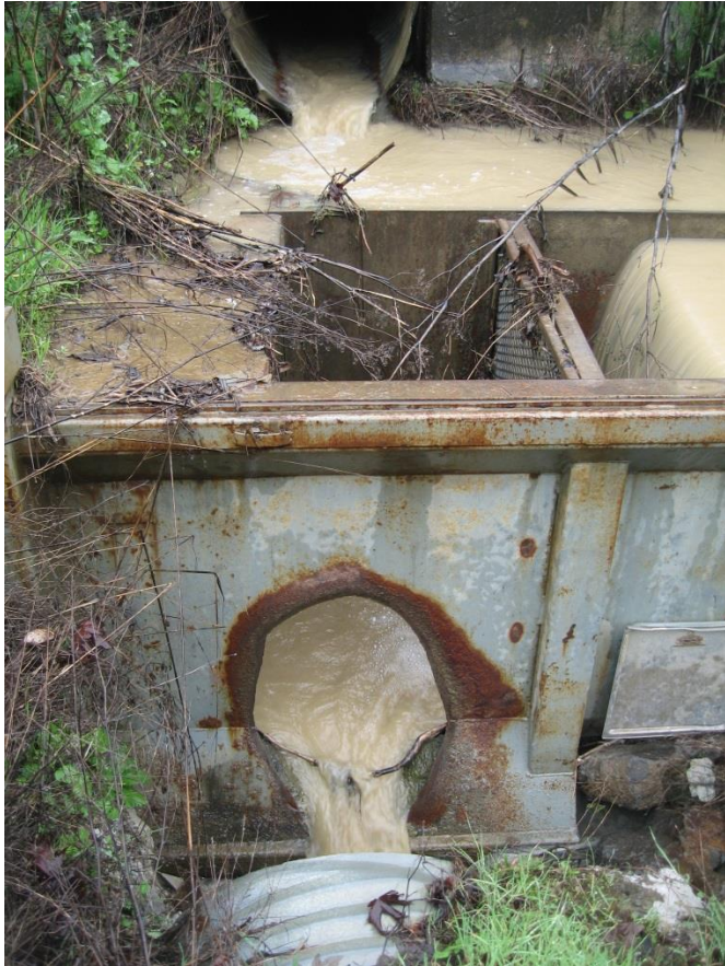
February 19, 2016 – Photo 1C. Point of discharge of turbid runoff to culvert that discharges into Mark West Creek. Paul Keiran, Regional Water Board staff photograph.
